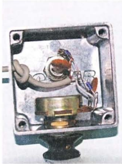
Photo 3: Showing the point to point wiring.
