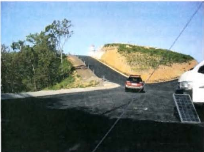
A view of Grassy Hill Lighthouse following recent road works.
