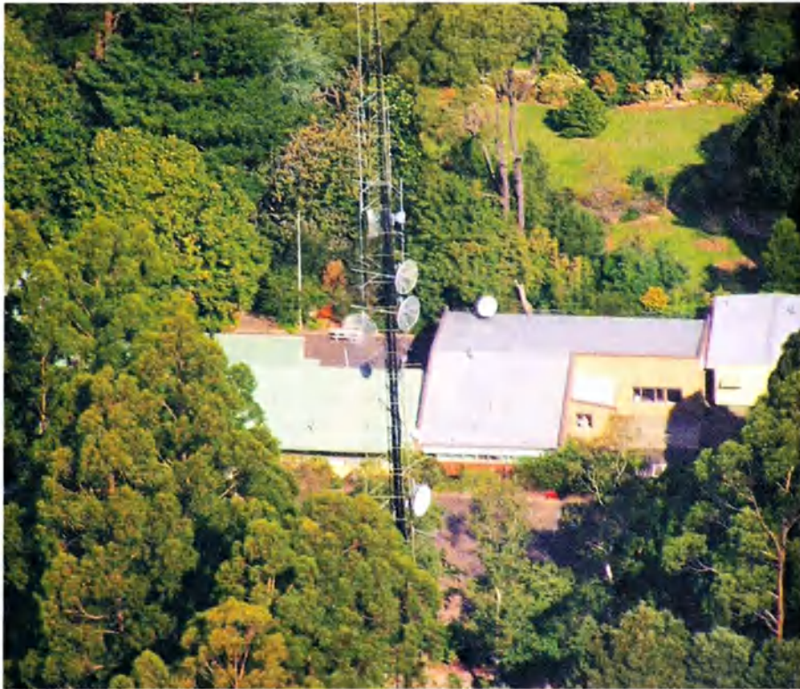
Photo 1: The VK3RTV repeater site.
