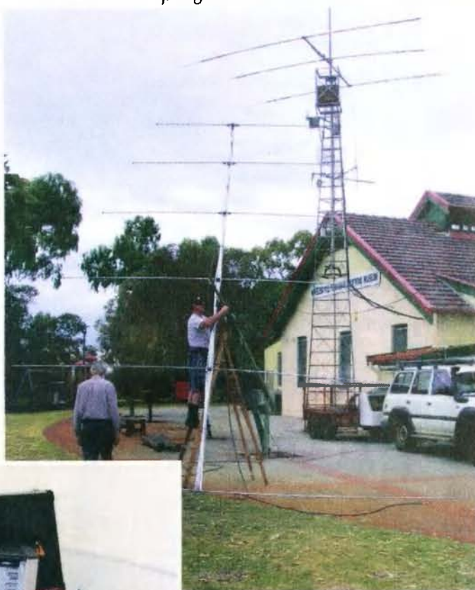
Above: Bob VK6KW working hard each day on improving our antennas – Installing 6el log periodic at Wireless Hill.
