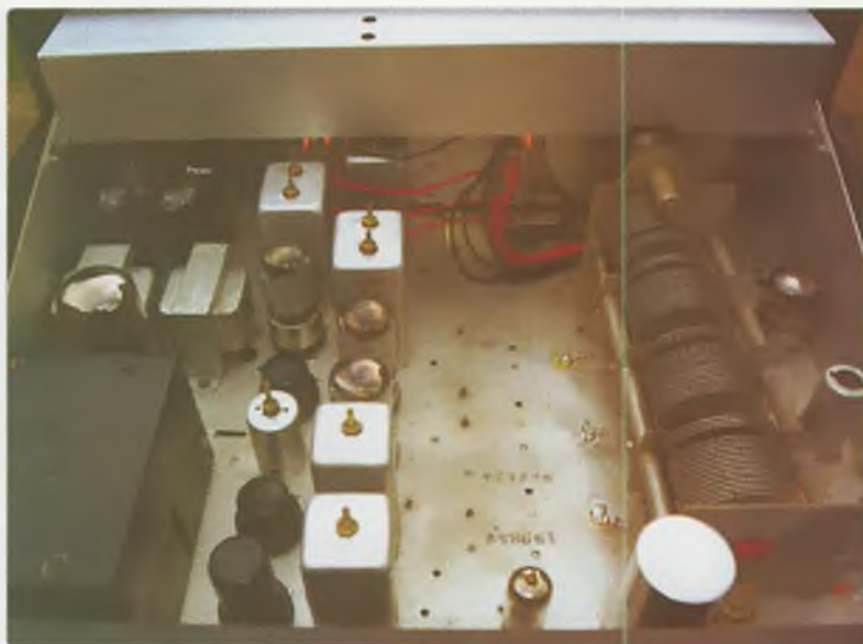
Photo 4: The top view of the chassis reveals the power supply and audio stages on the left, the two IF stages and detectors lined up through the middle and the front end RF sections on the right. Note the specially-built tuning gang that serves for the MF, HF and VHF bands.
