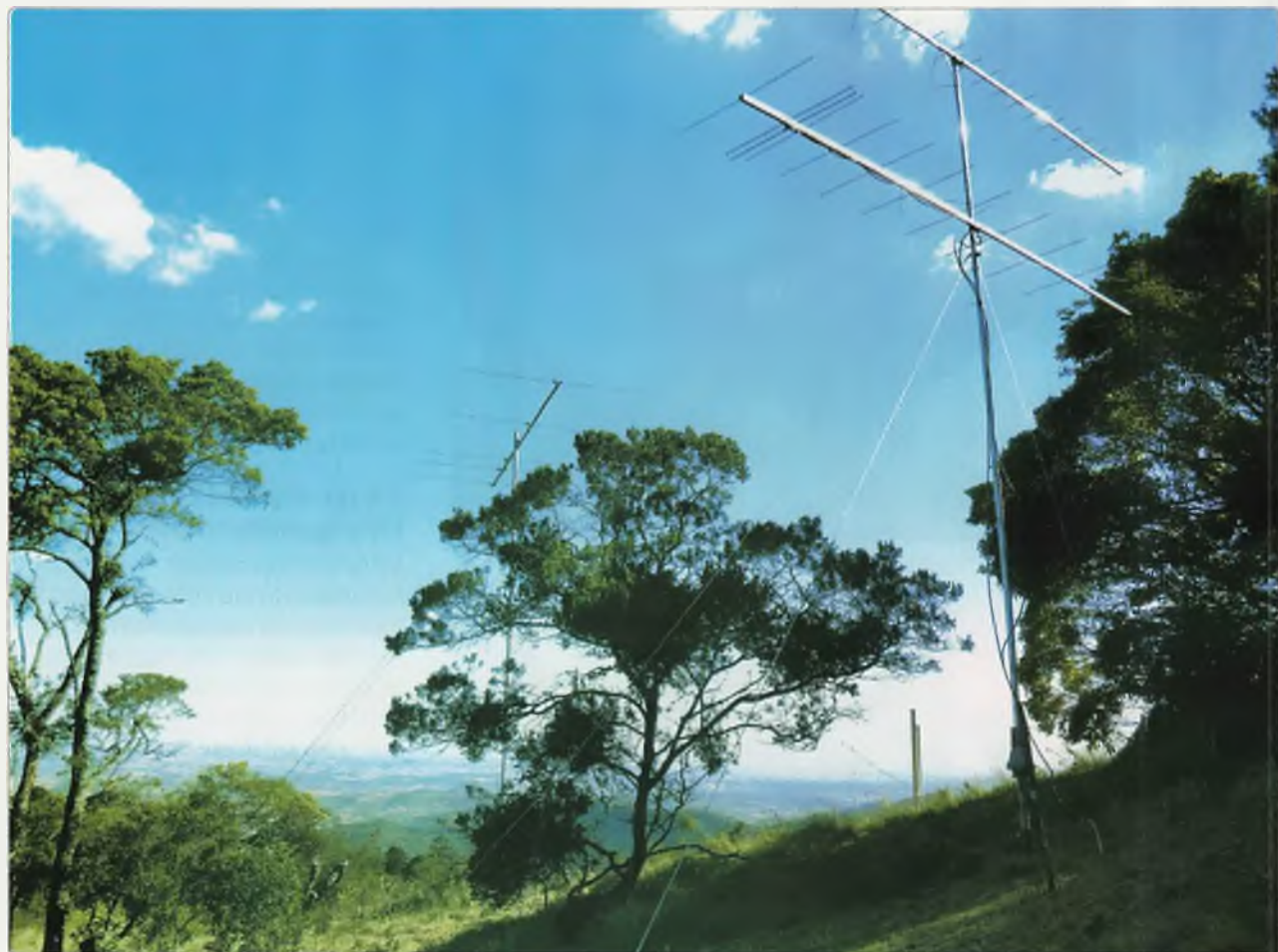
Photo 4: The Yagi arrays for 5m (on the left), on one mast, and for 2m and 70cm on the other mast, at right.
