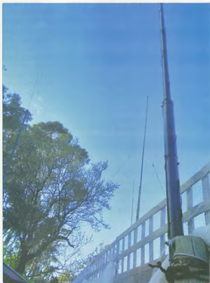
Photo 7. End view of three elements in-line, east to west.
