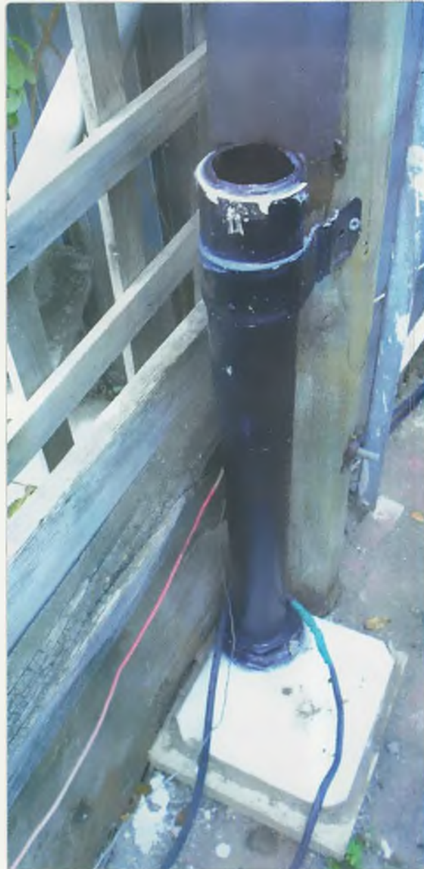
Photo 5: Black PVC irrigation riser as a ‘socket’, mounted on Teflon pad.
