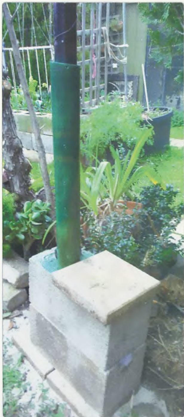
Photo 6. Concrete block base mount for element socket.
