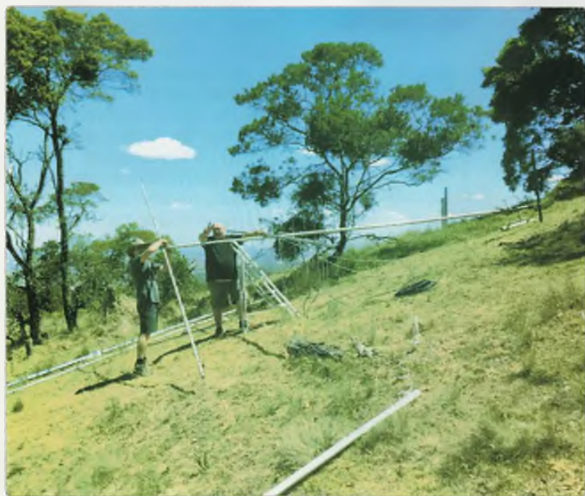
Photo 4: The Yagi arrays for 5m (on the left), on one mast, and for 2m and 70cm on the other mast, at right.
