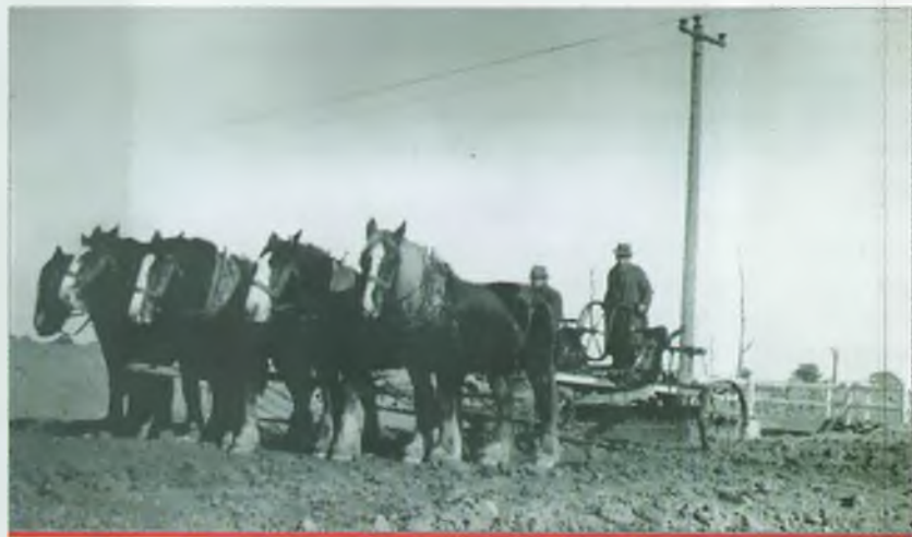
Horse power was used during Shepparton's construction. Here, horses and a grader are filling-in control cable trenches circa 1943 or 1944.
