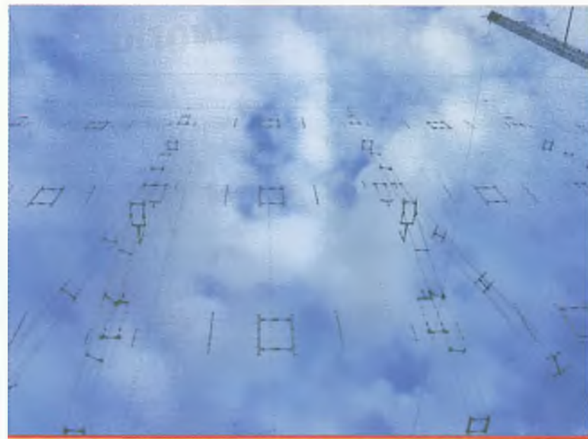
One of the curtain array antennas viewed from immediately beneath.
