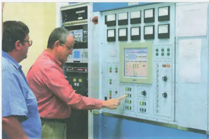
Radio Australia signs off. The final station manager, Nigel Holmes, turns off the last transmission from Radio Australia. The transmitter here was a Continental 418G AM-DRM (Digital Radio Mondiale) model.
