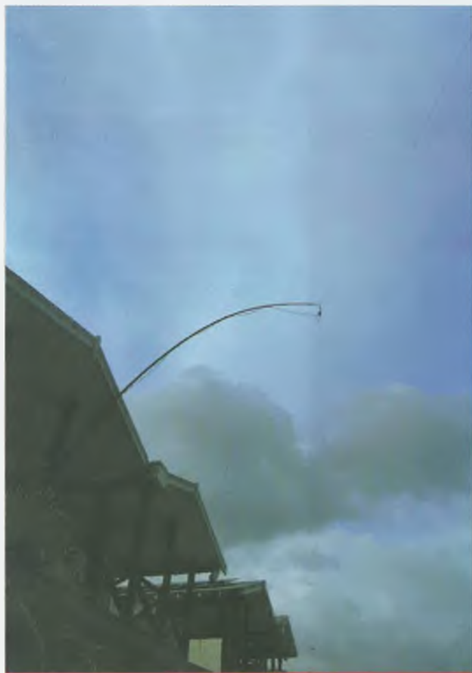
I lashed the squid pole antenna support to the accommodation's balcony railing.
