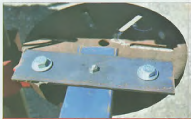
Figure 6. Securing the RHS tube.
