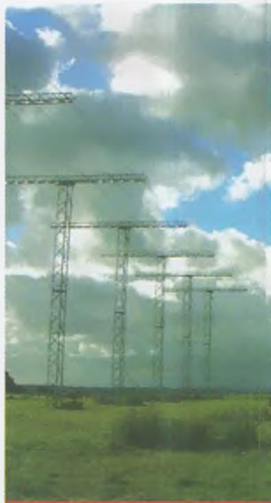
SuperDARN research installations feature arrays of wideband beam antennas. This photo shows a New Zealand installation. (Wikimedia)
