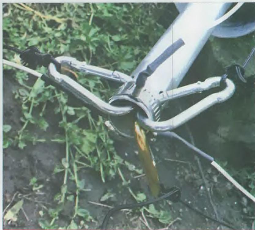
I used aluminium carabiners for strain relief with the capacitive hat.
