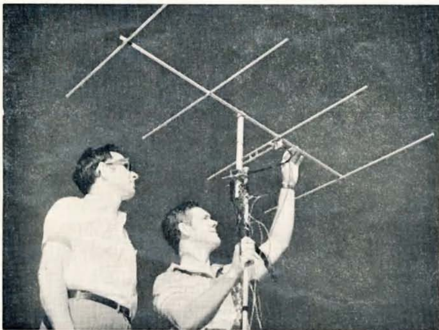
Bob Grummitt, VK4ZRG (left), and Bill Sebbens, VK4XZ, installing the 146 MHz. FM link antenna at Mt. St. John. This picture is of interest to those who have had poor results when trying to photograph antennas. This shot was taken at 10.30 a.m. using Kodak 32 A.S.A. Panatomic X film and an electronic flash. The camera was fitted with a 3-stop red filter which has had a startling effect on the blue sky.
