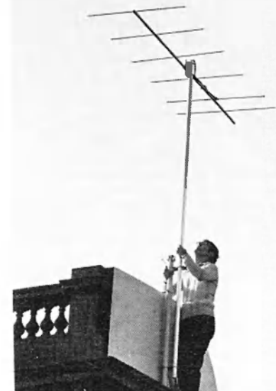
Les Janes VK3BKF installs a 2m antenna at Port Melbourne for Project ASERT.
