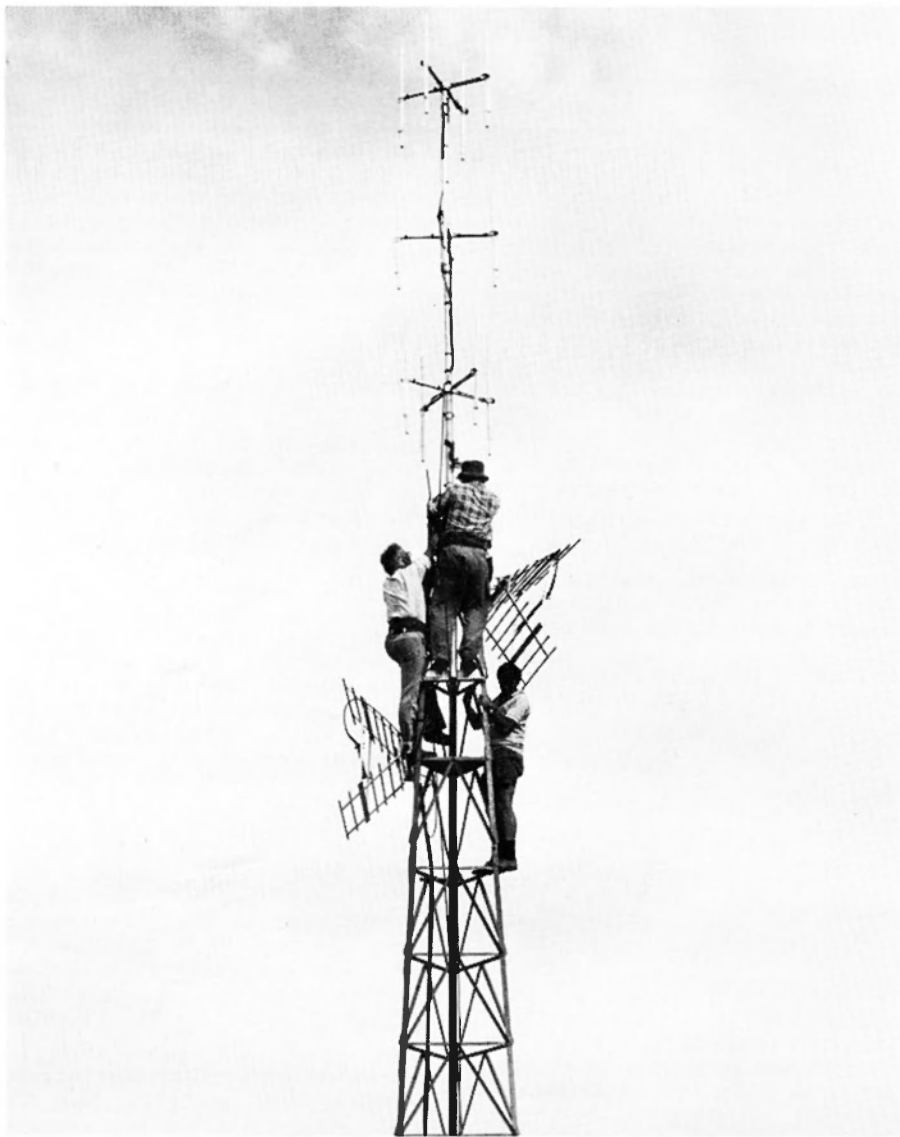
PHOTO 4: Reaching for the top on VHF! VK1 amateurs installing the ill-fated Mt. Ginini repeater installation on 12th February 1977. The original repeater antenna system featured 3 bays of 4 gamma matched dipoles fed quadrature (90° out of phase).
