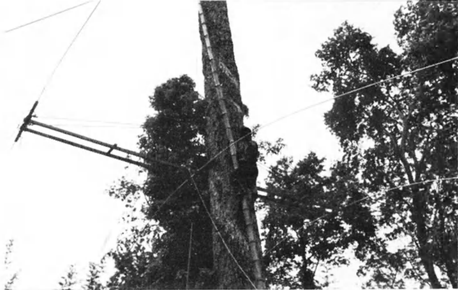
The homebrew 3 element yagi being erected for XZ5A.
