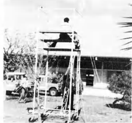
Mast with guy ropes about half way up.
