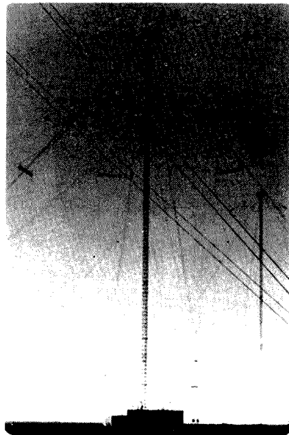
Tower Zero, U.S. Naval Base, Exmouth. 1274 ft. high, it has lift for two people inside. Centrepoint for all the rhombics.
