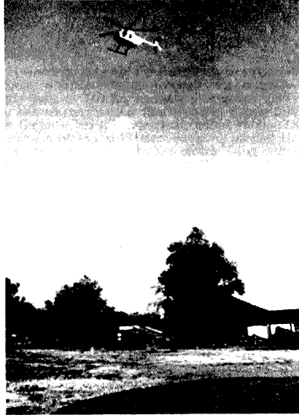
The first lift by the helicopter.
