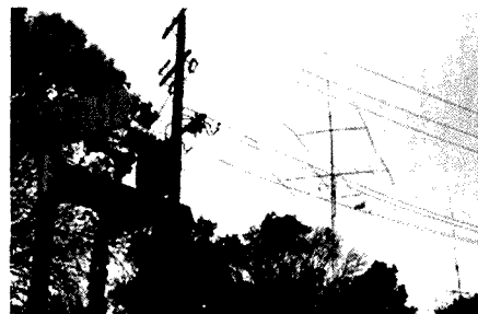
The Transformer which was replaced two years ago outside the VI2BVS QTH. In addition, all nuts and bolts were secured when the Transformer was revamped, and no problems have since been observed, especially during the intensive one month case-study. It is expected that a tightening of hardware, or cleaning of Disc Insulator Metal Parts and/or tensioning will cure the PLN at this case-study.
