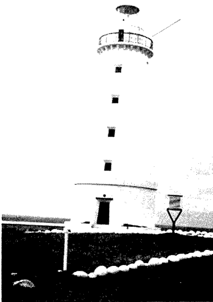
The lighthouse with the first jib on the top right of the house.
