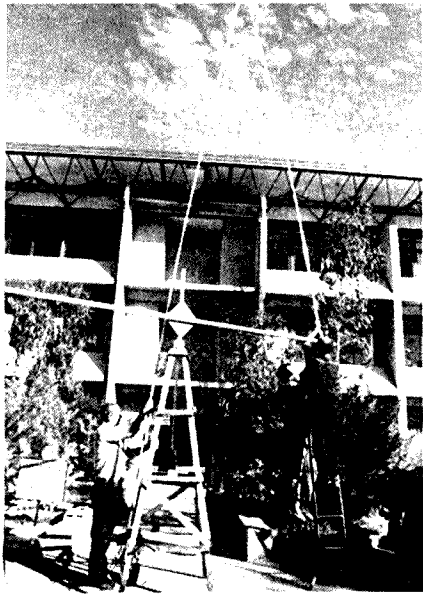
Erecting the Delta antenna for the RD Contest.
