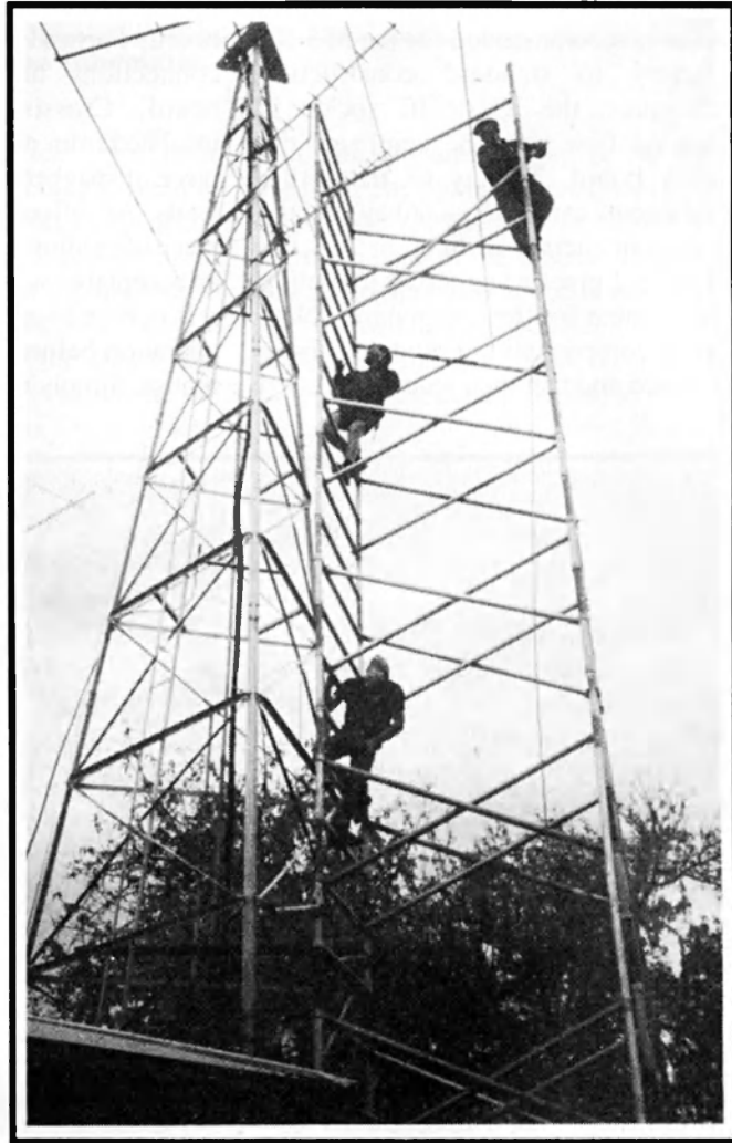
The instant scaffolding being erected.
