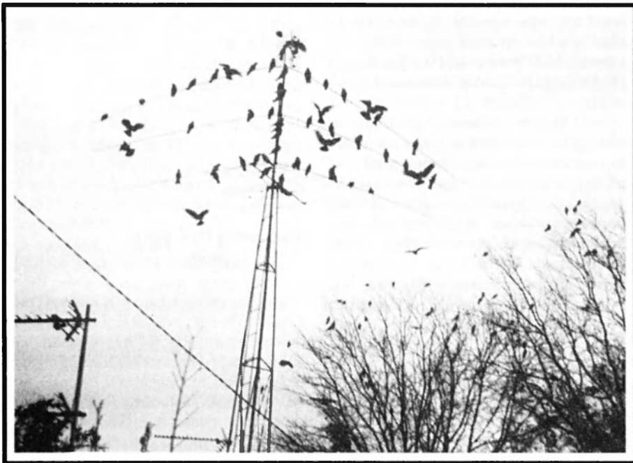
68 galahs perched on VK2BUE's 21 MHz Yagi beam elements (a frequent occurrence), which alters the horizontal into an "inverted vee".
