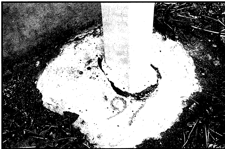
Photo 5 - Base of the steel post.
