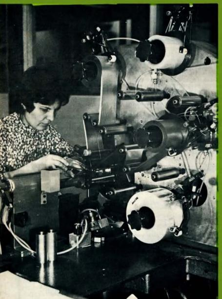
Despite a lot of talk recently that the component industry in Australia is finished, at least one factory in Melbourne is in full production of capacitors. This particular machine is winding metalised paper capacitors for the telephone industry. Photo: VK3ACA
