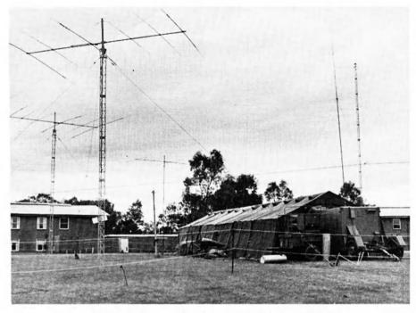
Antenna Farm at AX3SIG during exercise Ham Fest. Visible are 3 TH6DXX beams, 160Mx mast, whip antenna on Collins Mobile Communications Centre.
