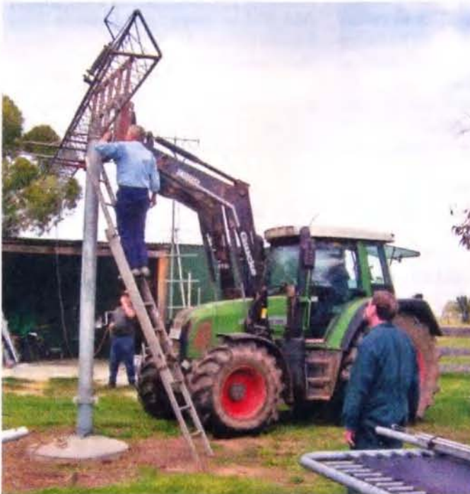
Photo 6: The lattice section being placed onto the in ground pole.
