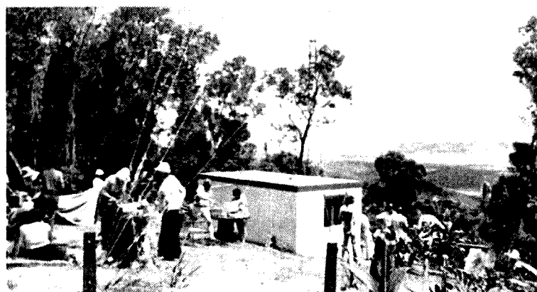
Official Opening, October 1978. Shack painted, tower up, and partying.
