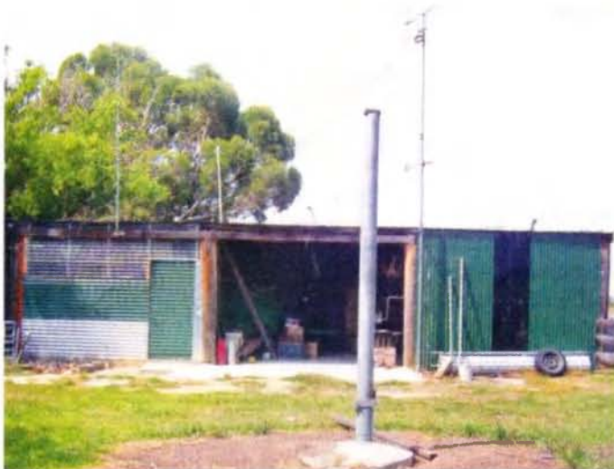
Photo 2: The tower pole in ground outside the shack, at Tinamba.
