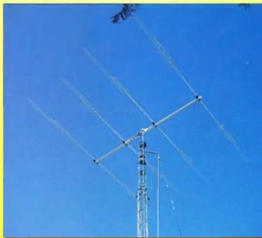
The nested two element quads for the six and two metre bands.
