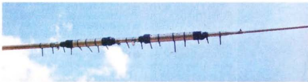
Photo 4: The traps as they appeared after the two pronged refurbishment was completed.
