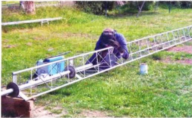
Photo 5: Welding the base plate to the tower.
