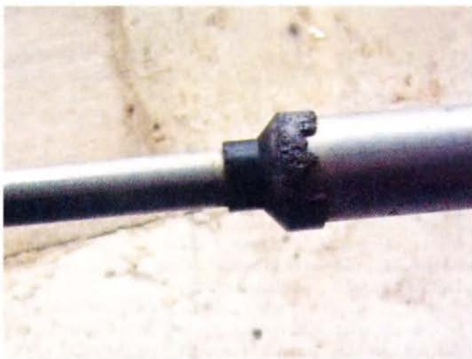
Photo 3: The TH6DXX traps before refurbishment.
