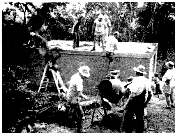
Above and below: 1976 Laying of the blocks for the Mt Goonaneman Repeater shack.
