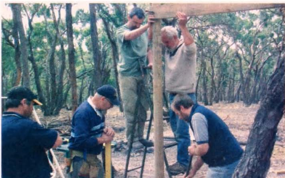
Dereel construction. Phase 1 of the alfresco area in progress
