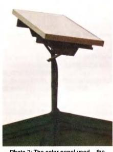
Photo 2: The solar panel used – the source of the power to replenish the batteries.
