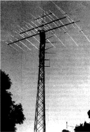
The 45 metre ex-SEC tower with the massive log periodic antennae erected by Bill VK3AMH and John VK3HW
