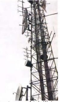
The antenna array of stacked Yagis can be made out amongst the many other antennas on the tower at the Mt Dandenong transmitter site.
