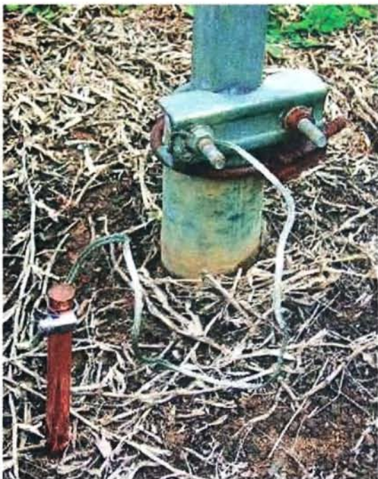
Photo 1: The earth stake at the base of the 10 metre high pipe mast.
