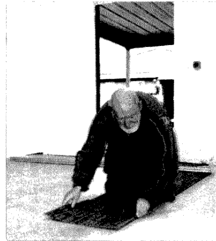
Photo 2: Barry VK5TW tiling at the 'Shack'.
