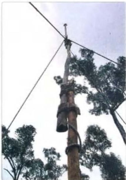
Photo 2: A mast built and erected by the Scouts for UHF CB communications back to base.
