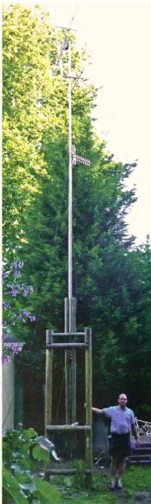
Photo 2: The completed and safer 11 metre antenna mast.
