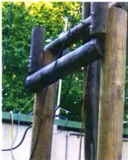
Photo 3: The 'U' shaped fulcrum at the top of the poles.
