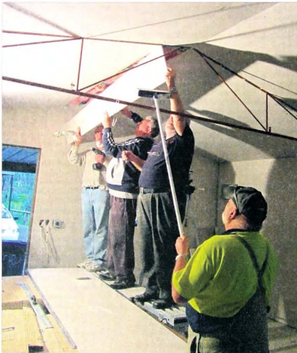
AHARS members hard at work on the Guide Hall refurbishment.
