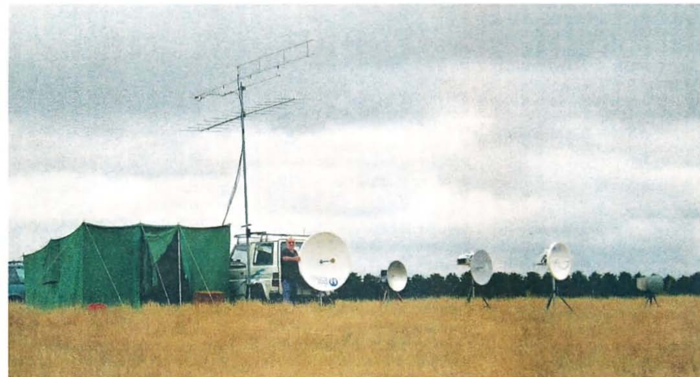
Photo 1: GARC Team LUMEG and their microwave installations.
