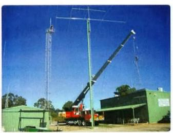
Photo 2: The principal antenna mover, the crane, in the operating position.
