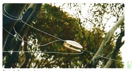
Photo 6: One end of the antenna wire supported by a tree.
