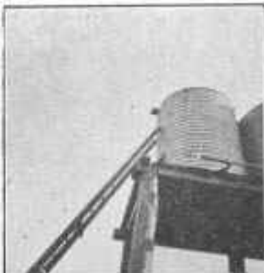
The Water-Tank-Aerial Tower at Bill's Hotel, Bateman's Bay.
