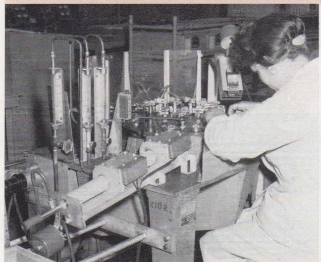
▲ Fig. 2. Twelve-head rotary machine for sealing glass tubes to cathode holders during manufacture of half-diodes. On right is a completely assembled half-diode.
