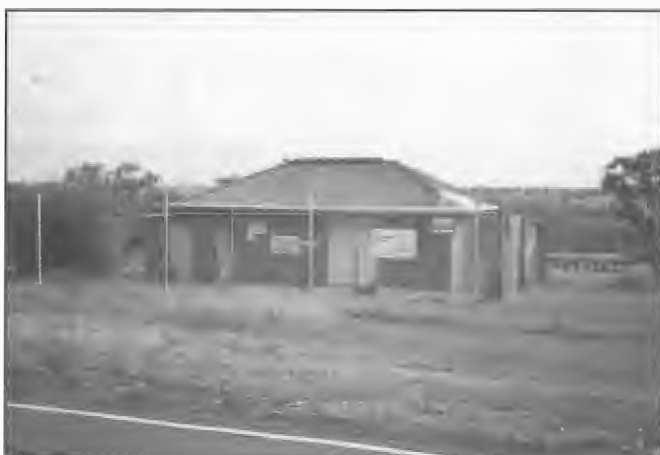
The 3RPH transmitter building Lower Plenty accommodating TBC type AM10KD 10 kW transmitter derated to 5 kW as main unit and STC type 4-SU-55 5 kW transmitter as standby unit. The station originally belonged to Commercial station 3KZ which established facilities on site and went to air in March 1956 with a 135 m lattice steel radiator. In 1971, a 54 m high standby radiator was erected. A standby diesel engine power plant located in a room on the left side of the building was installed in 1966.
