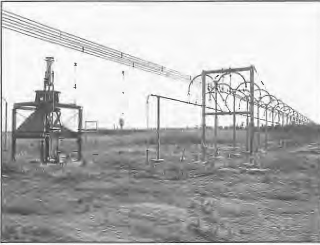
External type dummy load with water cooling system installed at Radio Australia Cox, Peninsula 1969. The 300 ohm dissipative line was constructed of 306 metres of 50 mm diameter stainless steel tubing through which water passed. The line had capability of dissipating 500 kW. It was damaged during Cyclone Tracy 1974 and dismantled.
