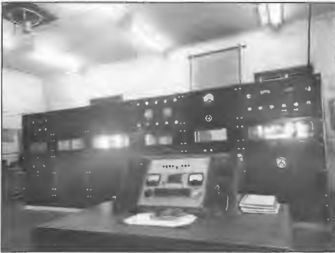
Transmitter 5CL Adelaide installed at Brooklyn Park in 1936. It replaced the AWA transmitter installed for Central Broadcasters Ltd original operators of the A Class station. The new transmitter provided 5 kW into the aerial. The final stage was a linear Class B amplifier using 4220C water cooled triodes. A motor generator supplied DC for the filaments of the water cooled valves. Ted McGrath was in charge of the installation.
