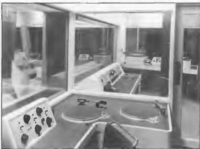
ABC studios Melbourne Show Ground circa 1948. Typical of post War facilities provided at similar Show Ground studios in major capital cities. Facilities included Announcer's console, technical control desk, disc replay desk with twin turntables and dual disc cutting equipment.
