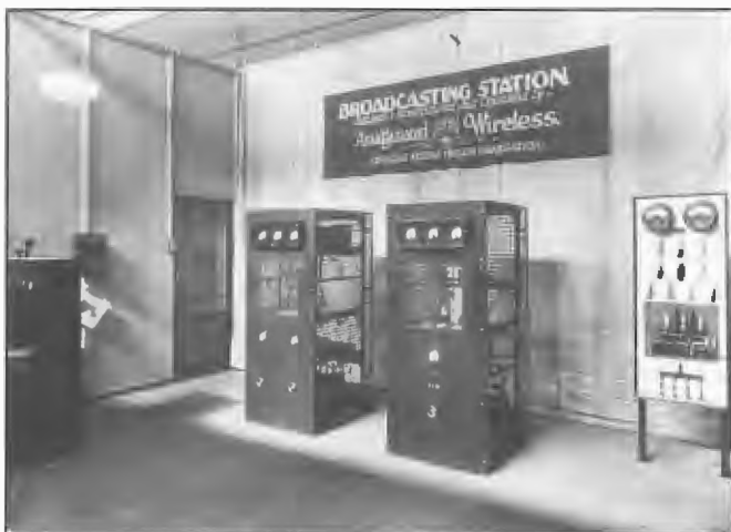
Broadcasting station 3EX designed and built by Amalgamated Wireless (A/Asia) Ltd and on display at the 'Made in Australia' Exhibition, Melbourne 1929. The exhibit was a complete station and was activated each evening to produce and transmit special programs of entertainment. Visitors could see the plant, operators and artists through large glass panels. Transmissions were conducted on 240 metres. The design formed the basis of transmitters being planned for commercial broadcasting during the following year, 1930, during which 12 Commercial stations were commissioned.
