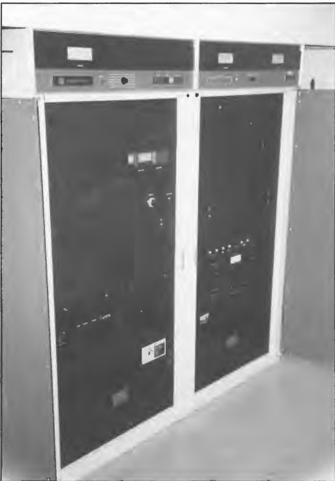
One of a pair of 10 kW Harris MW10 transmitters used from September 1990 for 4RPH Tingalpa near Brisbane and operating on 1296 kHz. The transmitters derated to 5 kW each were originally part of 4BK facility until that station transferred to the FM band. Harris transmitters are manufactured in USA by Harris Corpn and distributed in Australia by Comsys Pty Ltd.
