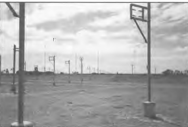
Open wire transmission lines at Brandon, North Queensland associated with MF and HF services. The 200 ohm six wire line is part of the MF NBS 4QN facility while the 300 ohm four wire line is part of the Radio Australia HF service. Masts in the background support HF curtains.
