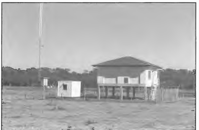
Typical of measures at some transmitting sites to prevent interruption to service in times of flooding of the site. The station operated by 4RPH since 1990, was originally operated by 4BK. Transmitter building, aerial base insulator and aerial coupling unit are mounted above expected flood water level. The mast is one of a directional pair.
