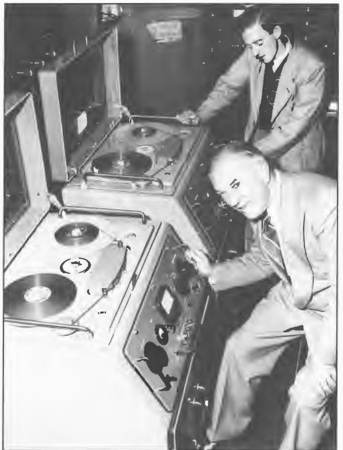
EMI reel-to-reel tape recorders in service at 3AW Melbourne 1956. Announcers Norman Banks and Graham Evans observing the units. These types of recorders were widely employed at ABC and Commercial studios for many years. One of the earliest installations of this static recording equipment was provided at Parliament House, Canberra for use by ABC programmers.
