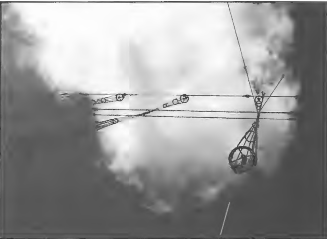
Some of the conically shaped dipole elements of the five dual plane log periodic aerial systems provided at Radio Australia Cox, Peninsula 1969. The vertically polarised aerials all covered the frequency range 5.95 MHz to 26.1 MHz and were fed by 300 ohm open wire balanced transmission lines. Contractor's Engineer, Ross Burbidge.
