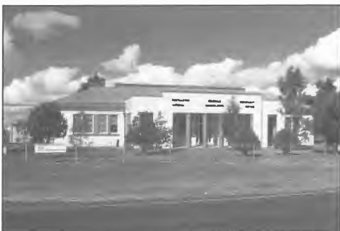
Transmitting station building 4QS Dalby, erected 1939. First Officer-in-Charge Harry Conway.
