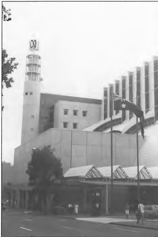
The Ultimo Sydney studio building of the Australian Broadcasting Corporation opened during June 1991. The entire building is constructed on massive piles socketed into bedrock to render the building as insensitive as possible to vibrations from nearby road and rail traffic. Each studio is a separate box-like construction within the building. Cost of the project was $150 million.
