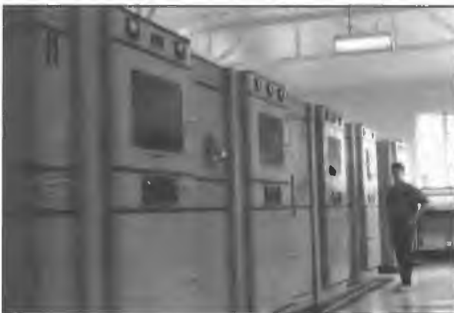
VLM 10 kW transmitter type STC type 4-SU-12A installed January 1951 at Bald Hills for HF Inland service and still operational when service closed down during December 1993. Operational frequency was 4929 kHz. Beyond David Sanderson standing near the VLM transmitter, is 2 kW unit used as standby for 4QG (4RN).
