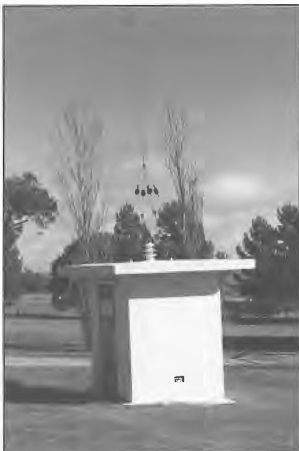
Alexanderson type aerials commissioned at 5CK, 2CO and 6WF in the early 1930s employed two tuned down leads at the ends of the horizontal
