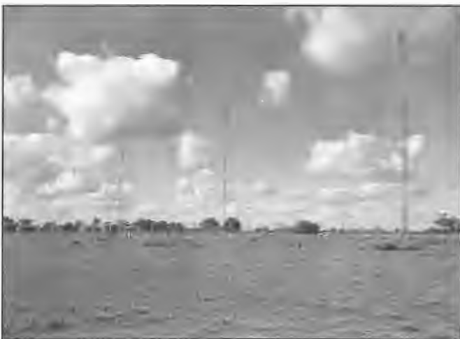
Single frequency curtain aerials provided at Radio Australia, Shepparton 1945. Nineteen directional arrays were supported by 14 guyed lattice steel masts each 66 m high. A switching system provided for reversing the direction of radiation of some aerials and also for slewing some in the horizontal plane. Engineer, Jim Wilkinson was associated with lining up and commissioning the systems.
