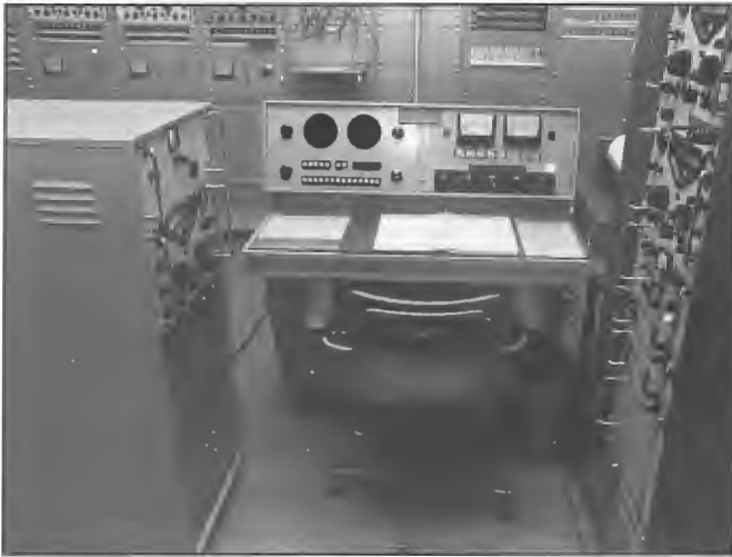
A program reception and control position at Receiving Station, Cox Peninsula, installed 1969 to provide off-air programs from transmitters at Shepparton, Victoria, for rebroadcast by 250 kW Radio Australia transmitters located at another site on the Peninsula. Booth program and control positions were equipped with Racal RA117-C2 receivers with RA98C-1 independent sideband adaptors set up for dual diversity reception mode. A spare position was set up in the receiver hall. The facility was closed down in 1974 when direct circuits to ABC Radio Australia, Melbourne became available. Installation Engineer, Brian Woodrow.
