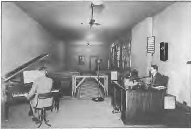
Studio at 5AD Adelaide. The 21 m by 6 m studio walls and ceiling were lined with Celotex. The station in the city centre, commenced operation with a 300 watt transmitter on 2 August 1930. Harry Kauper formerly Chief Engineer 5CL, designed the technical facilities.
