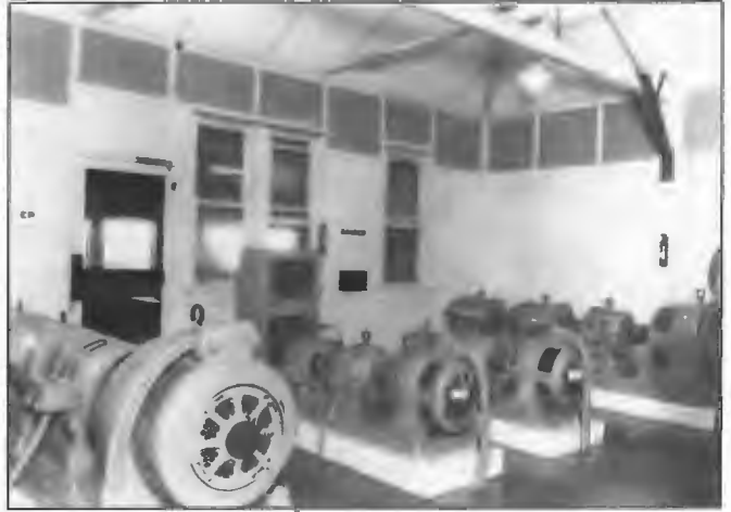
The 4RK Rockhampton machine room 1931. Power requirements for the 2 kW transmitter were provided by duplicated motor generator sets. High tension supplies were generated by two double wound generators driven by a common motor. The filament and bias supplies were provided by separate units. The machine room also contained the water cooling pumps. Station 2NC Newcastle had a similar installation.
