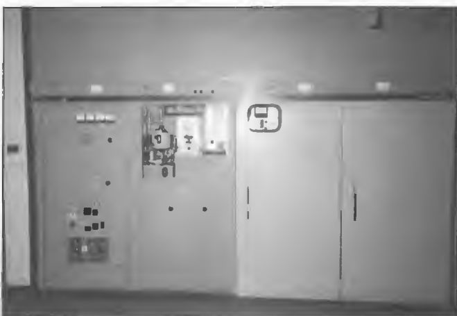
100 kW Harris/Gates transmitter installed Radio Australia, Carnarvon 1976. It employed pulse duration system of modulation.
