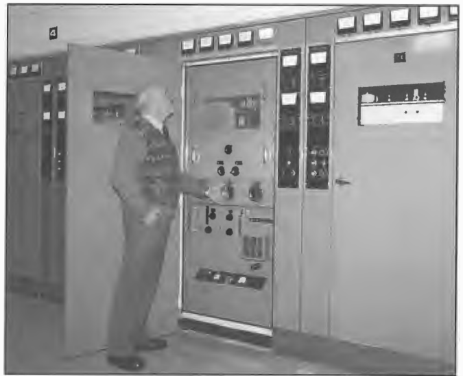
Max Fowler, last Officer-in-Charge at Lyndhurst before closure 1987 adjusting one of the STC 10 kW transmitters. In the 1960s, eight new 10 kW transmitters were installed.
