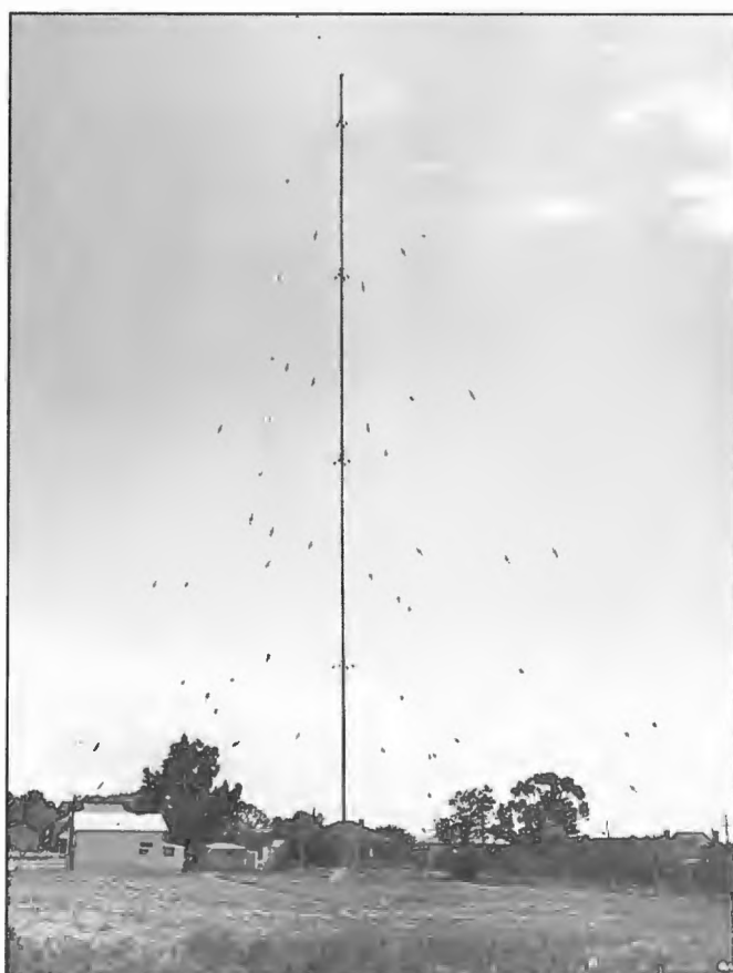
Tubular 50 m high radiator installed at 5MU Murray Bridge 1949. It replaced the original six wire flat top type installed when the station was commissioned in 1934 by Frank Miller.
