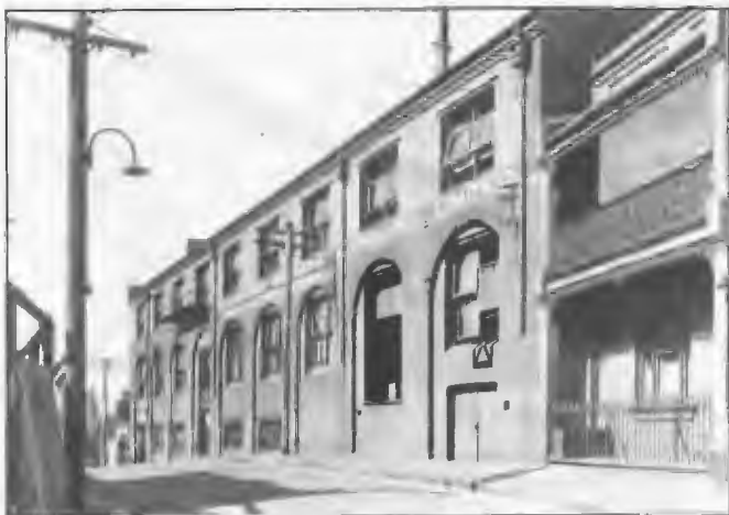
Amalgamated Wireless (A/Asia) Ltd, Radio-Electric Works at Knox Street, Darlington. The premises were occupied in 1922 when it became evident that the Clarence Street premises would not meet the future needs of the company with the introduction of broadcasting being planned by the Government. The Knox Street factory became the key centre in the production of broadcast transmitters, home receivers, ship's wireless apparatus and a multitude of radio components.
