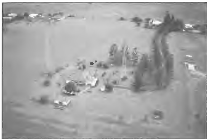
View of 4RK Rockhampton taken 1987 from the station 128 m high radiator showing the original building and aerial provided in 1931. In 1998 the aerial was still in service as a standby. The residence of the station Officer-in-Charge is at the end of the tree lined driveway. The trees were planted by Harry Conway the first OIC.
