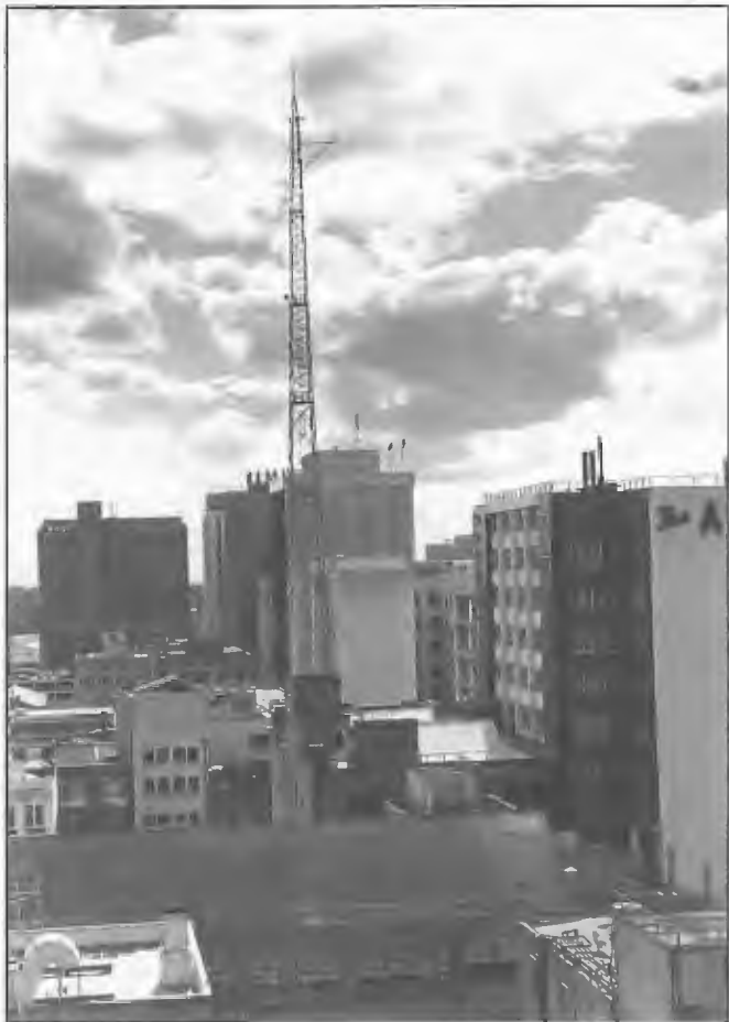
Self-supporting 60 m tower on roof top of Perth GPO employed as the radiator for 6WN which went to air on 12 October 1938. The feeder linking the 500 watt transmitter to the aerial was an 80 ohm concentric type. During the War years, the tower was dismantled and the transmitter shifted to another site.
