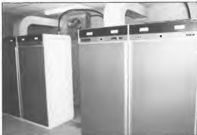
The 5 kW Harris transmitters commissioned for 3EA Melbourne on 26 January 1980. They were located at Craigieburn and fed a 61 m high directional aerial system. Neil McCrae was in charge of the project.
