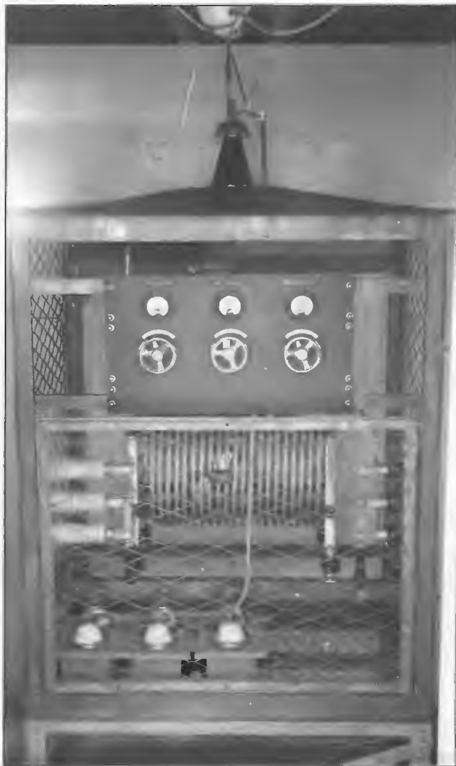
Aerial coupling unit 5DR Darwin 1963, showing typical components for a 2 kW station. Meters enabled measurements to be made of transmission line, aerial and network circulating currents. Knife switches allowed line and aerial to be earthed during maintenance activities. Installation Engineer, Joe Brady. Station call sign was later changed to 8DR.
