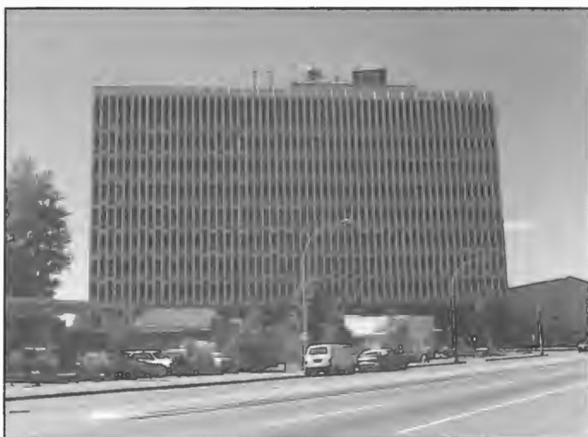
ABC administration and studio building Collinswood, Adelaide. The 5CL/5AN studio facilities were transferred from Hindmarsh Square into the Collinswood building on 13 October 1975. The building became the ABC headquarters for ABC FM Stereo when the service began in 1976.
