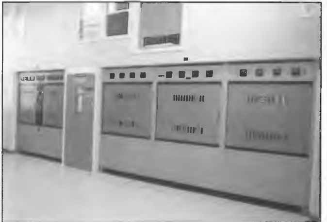
AWA 10 kW BTM10J standby transmitter (left) and 50 kW AWA BTM50 main transmitter at 2CR Cumnock. The station began operation in 1937 with an STC 10 kW transmitter. In 1963, a 50 kW AWA transmitter was installed and was the only such transmitter installed in Australia. When originally installed, it employed English Electric AR63 mercury arc excitrons of a single anode mercury pool type in the main rectifying system. The transmitter was operational until January 1994 when it was replaced by a Nautel solid state model.
