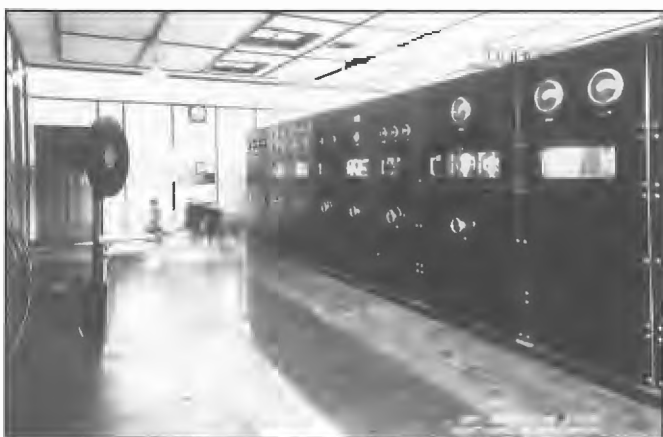
(a) The 6WF Perth NBS transmitter after commissioning on 14 December 1932. Tests showed it produced an unmodulated carrier power into the aerial of 3.6 kW giving an overall efficiency of 15%. This was the first time the PMG's Department had undertaken the entire design, construction and installation of an MF broadcasting station.
