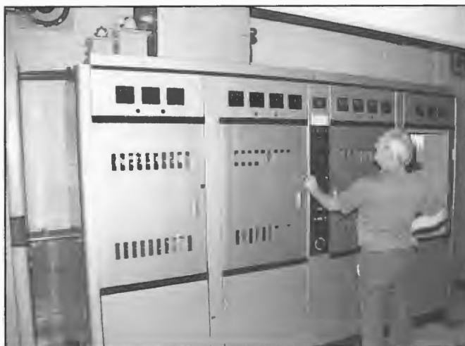
Graeme Wilmot, Officer-in-Charge, 7ZL/7ZR Hobart adjusting the 7ZL AWA BTM10 transmitter which was installed during 1958 sharing a dual frequency radiator with 7ZR. A directional radiator was put into service in 1964.
