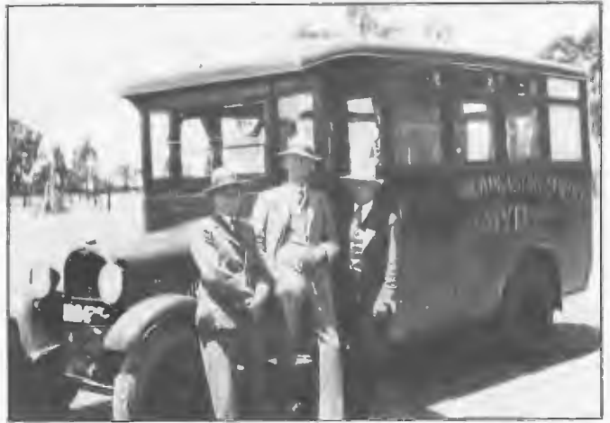
The studio A Model Ford van used with mobile station 3YB October 1931 to October 1932. The studio facilities included record cabinet, two turntables and Reisz carbon microphone. The van was painted scarlet with '3YB Mobile Broadcasting Service Pty Ltd 262 metres' in gold lettering on the sides. L to R: Bert Rennie, Business Representative and power plant operator; Vic Dinneny, Manager and Announcer and Bert Aldridge, Chief Engineer.
