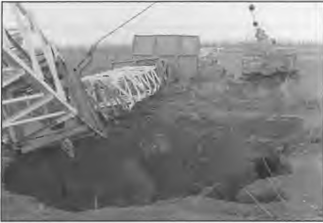
Extent of damage from Cyclone Tracy 1974 to one of the aerial support masts Radio Australia, Cox Peninsula. The wind pressure on the structures was so great that concrete anchor blocks were ripped out of the ground. It was 1984 before the station was fully rehabilitated. Station Engineering Manager when the cyclone struck was Max Chadwick.
