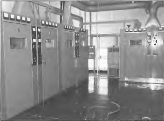
Three STC type 4-SU-48B 10 kW short wave transmitters at Radio Australia, Brandon. The transmitters had previously been installed at Lyndhurst in the late 1960s but on closure of that station were transferred to Brandon in 1989. Engineers associated with establishment of the station HF facilities included Janis Ozolins, Richard Womack and Doug Sanderson.
