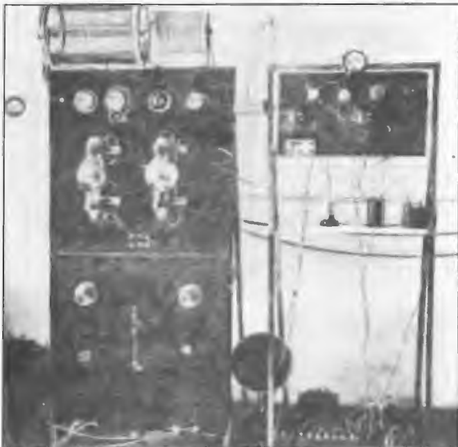
The original A Class station 5CL Adelaide commissioned on 20 November 1924 for Central Broadcasters Ltd on the roof of the Grosvenor Hotel. Input to the final stage was 175 watts. Don Gooding was in charge of operations.
