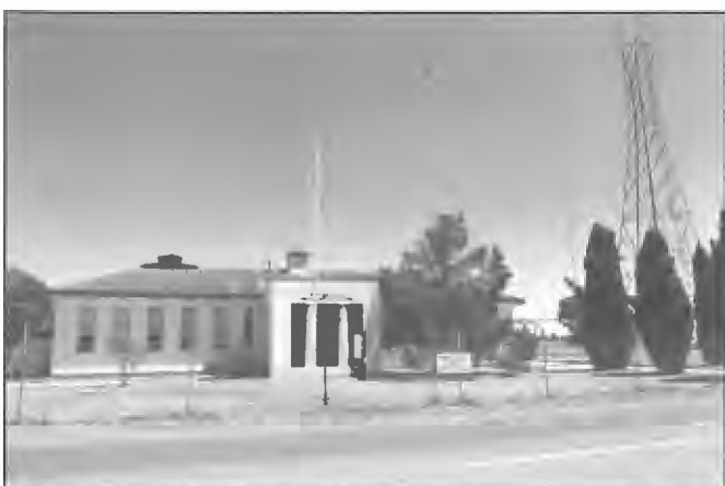
Transmitting station building 3WV Dooen, erected 1936. First Officer-in-Charge Stan Hosken.
