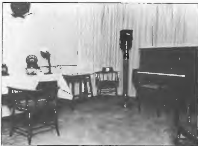
No. 2 studio 7ZL Hobart 1936. Facilities included condenser microphone on pedestal, WE double button carbon microphone and wall-mounted RCA loudspeaker for monitoring. These facilities were somewhat behind the times compared with ABC studios on the mainland during the period.
