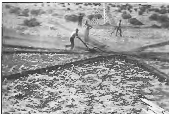
Before the advent of the mole plough for laying copper wires for a radial earth mat for a vertical radiator, trenches were either dug by hand or excavated by using an agricultural type plough pulled by a horse or truck. After laying the wires in the trenches by hand the soil was backfilled using a scraper, again pulled by the horse or truck.
