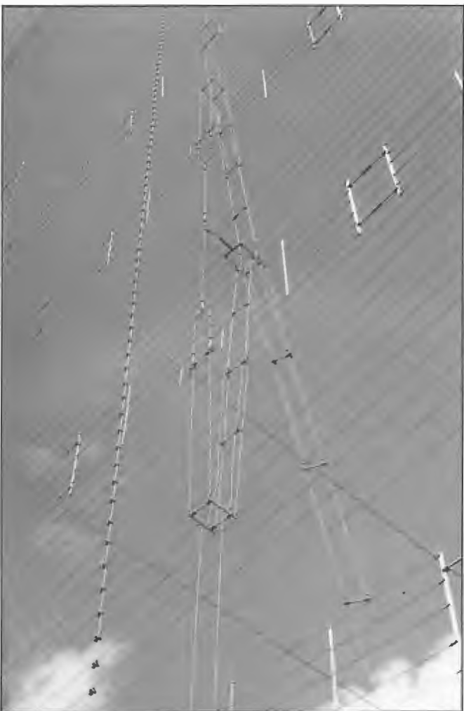
TCI Model 611 curtain aerial system installed at Radio Australia, Cox Peninsula 1984. The radiator assembly used three 2.8 mm diameter/alumoweld wires twisted together with the vertical support cables being stranded wires of overall 6 mm diameter. The feeder line transformer section used 12 mm and 6 mm diameter stranded cables. Reflector screen wires comprised aluminium wires suspended by 6 mm diameter stranded vertical bearer cables. Transmission from the station ceased on 30 June 1997 and the station placed in a caretaker mode using maintenance staff.
