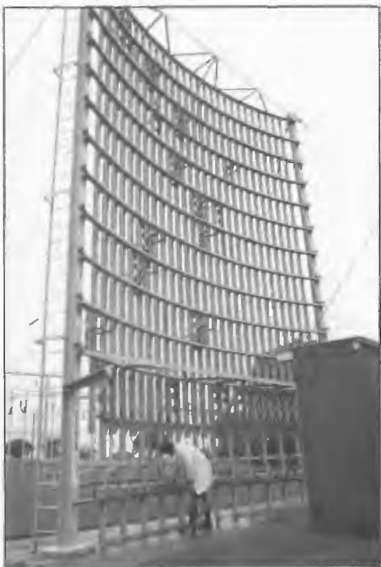
The 128 m sectionalised and top loaded radiator at 4RK Rockhampton erected 1954. It replaced the original four wire flat top aerial which had been in service since July 1931 when the station was commissioned. As at 1993, the original aerial was being used as a standby aerial. The new radiator was the first of the type installed in Regional Queensland. Commissioning Engineers, Mick Hall and Frank Sharp.
