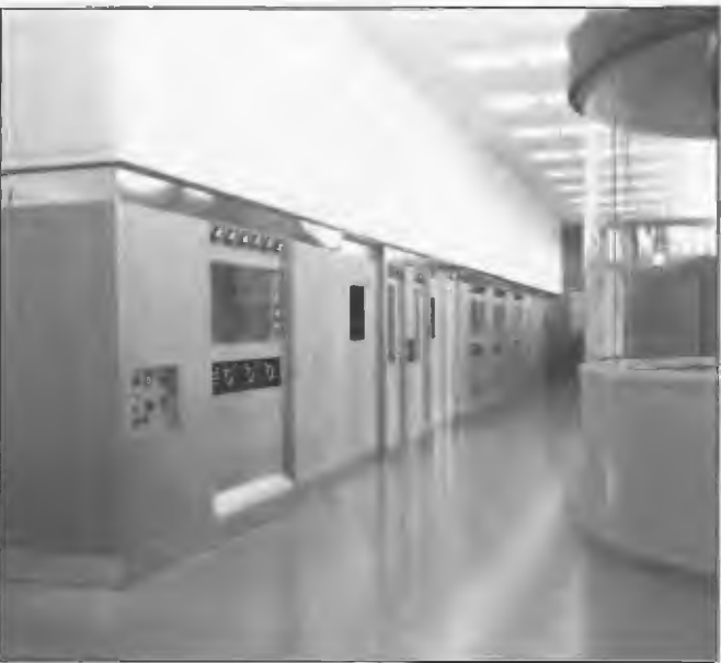
Transmitter Hall, NBS station Hamersley near Perth circa 1962. Transmitters comprised (left to right): 10 kW STC type 4-SU-64 main, 2 kW Philips type 1956 standby both for 6WN (later 6RN); 55 kW STC type 4-SU-38B main and 10 kW STC type 4-SU-64 standby, both for 6WF.
