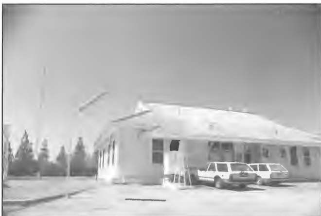
Transmitting station building 5CK Crystal Brook, erected 1932.
