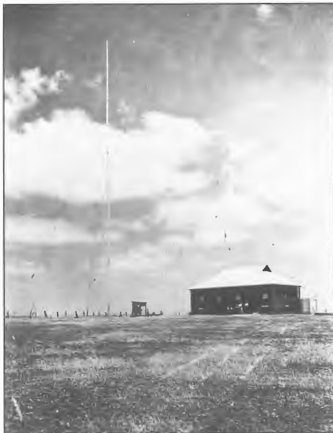
Six wire cage aerial at 5PI Port Pirie supported by two 41 m Oregon pine masts, 1934. It was an Alexanderson type with each end being tuned via variometer. Years later when it was dismantled, the Oregon masts were cut up and used as masts for small boats.
