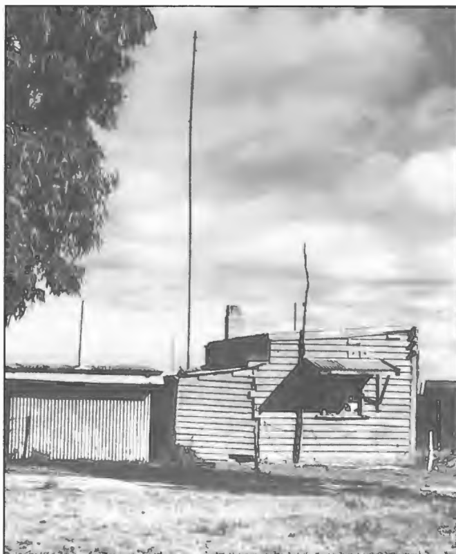
The original transmitter building at Lyndhurst near Melbourne in 1928 when the PMG's Department established an experimental HF transmitter on site. Transmissions were conducted 2-3 hours daily and beamed to Northern Australia. The transmitter provided 600 watts into the aerial on a frequency of 9580 kHz.
