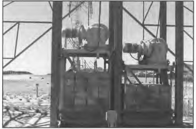
All four curtain aerials at Radio Australia, Carnarvon installed in 1975 were supported by counterweighted catenary ropes which were wound on to electric winches forming part of the counterweight. The winches allowed the curtains to be lowered to the ground for maintenance purposes and to be later raised to their correct operating positions. Carnarvon was the only station in Australia fitted with this facility.
