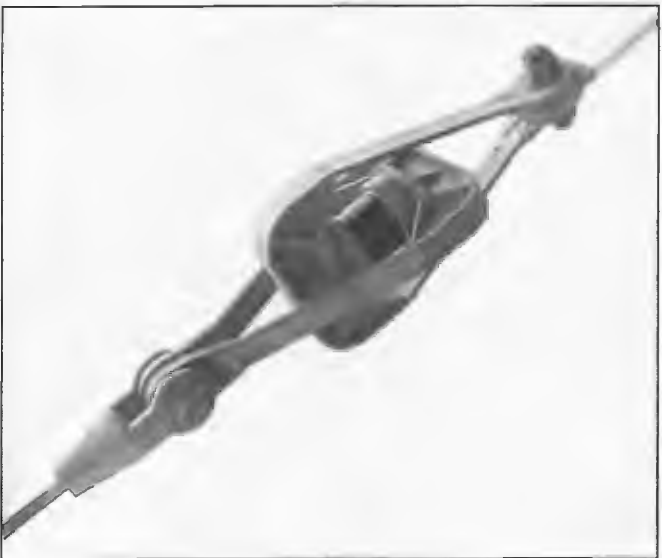
Guy insulator of the type installed at 5CL/5AN Pimpala and 5CK Crystal Brook 1961. The steel work was made in Australia but the porcelain insulator was manufactured in Japan. Insulator and steelwork were replaced by new designs in 1992.
