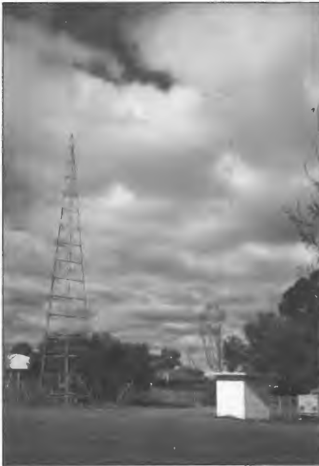
T type flat top aerial 22 m high using square section cage feeder at National station 5MG Mt Gambier. The station was commissioned on 26 September 1955 using main and standby 200 watt Philips transmitters. A PT29M coaxial feeder linked the transmitter to the Aerial Coupling Unit. Murray Higgins was Divisional Engineer-in-Charge of the installation. Station Officer-in-Charge, Bill Legg.
