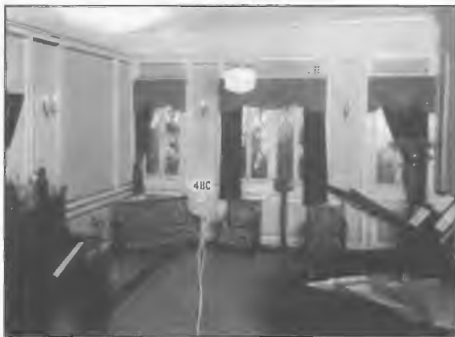
One of the 4BC Brisbane studios in the Wintergarden Theatre, Queen Street, Brisbane circa 1938. The Reisz microphone was typical of those used in other studios. Curtains covered the leadlight windows during a broadcast. Sound absorber panels were fitted above the windows and on the ceiling.
