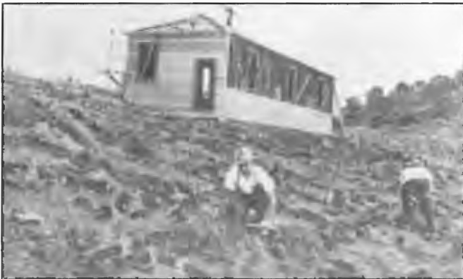
Erection of the 7ZL Hobart transmitter building and installation of earth mat at a site known as Radio Hill, December 1926. On 3 March 1926, the station was taken over by Tasmanian Broadcasting Pty Ltd from Associated Radio Company of Melbourne who held the original licence. Station Construction Engineer Donald Macdonald.
