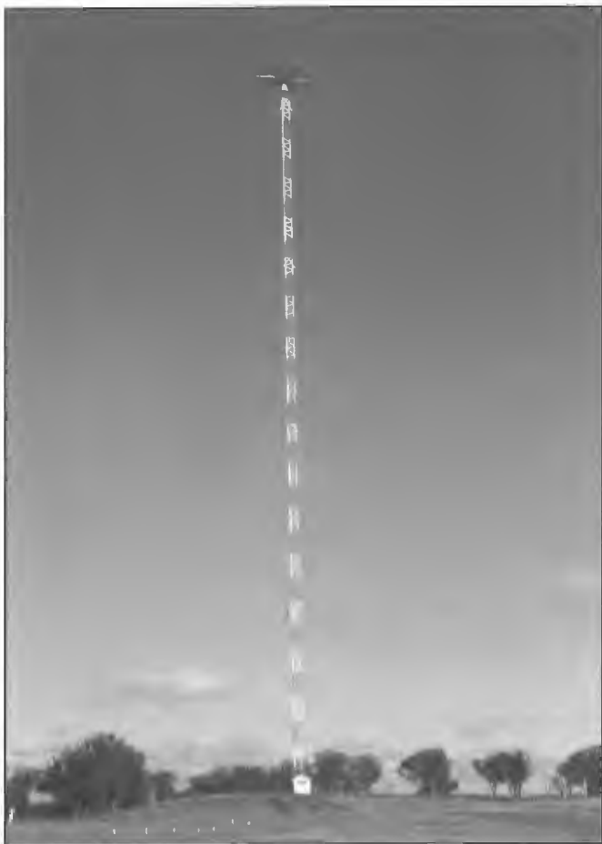
The 198 m lattice steel armature top radiator installed at 2CR Cumnock in 1937 and still in operation in 1998. The design was prepared by PMG's Department Research Laboratories in the mid 1930s and installed at many NBS stations. The horizontal armature is insulated from the vertical section and electrically connected via an inductor. The armature and inductor combination act as a termination equivalent to many metres of mast height. Alec McKenzie was responsible for design aspects.
