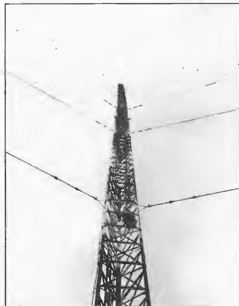
Typical lattice steel guyed omnidirectional radiator employed at Commercial stations in the 1950s. This 130 m radiator guyed at six levels was erected for 3SR Shepparton in 1956 at a site 12 km east of the town. It was fed by a 2 kW AWA transmitter operating on 1260 kHz. Chief Engineer was Ray Jenks. The radiator remained in service for 30 years until a new 130 m structure was commissioned in 1986 at another site following expiration of the lease at the old site.
