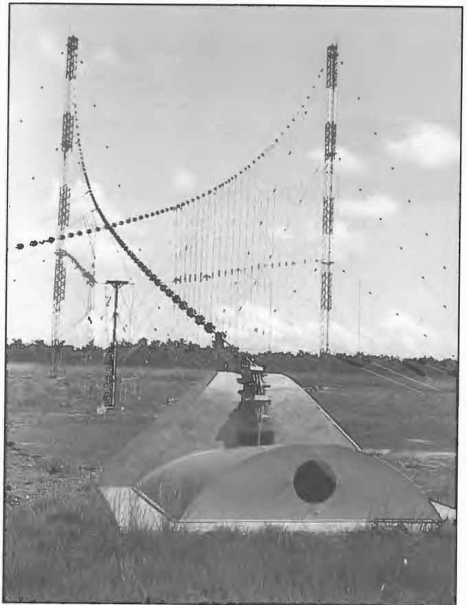
One of two dual plane log periodic vertically polarised aerials installed at Receiving Station, Cox Peninsula 1969 for off-air reception of programs originating in Victoria for rebroadcast by Radio Australia transmitters 16 km away on another site on the Peninsula. The aerials beamed on Shepparton were spaced 10 wavelengths apart at the lowest operating frequency. Signals were taken to the receiver hall equipment via an above ground rigid balun transformer line and a buried coaxial cable. The system was decommissioned during 1974 when direct program lines to ABC Radio Australia studios in Melbourne became available. Contractor's Engineer, Ross Burbidge.
