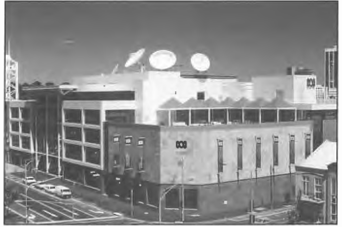
The Australian Broadcasting Corporation Southbank building officially opened on 5 November 1994 by Prime Minister Paul Keating. It caters for ABC Melbourne staff associated with 3LO, Radio National, ABC Classic FM, JJJ, Regional Radio, Radio Australia, Melbourne Symphony Orchestra and technical support services including a range of satellite services.
