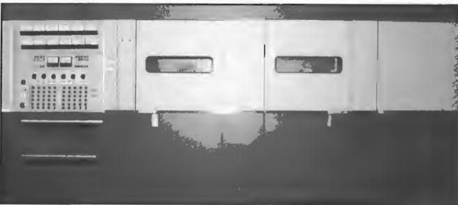
Continental Electronics transmitter type 418D-2 installed at Katherine, Tennant Creek and Alice Springs to provide service to Northern Territory using vertical incidence transmission. The 100 kW transmitters were cut back to provide 50 kW to the aerials. They were commissioned during 1986 and operate in the 60 metre band during the day and in the 120 metre band during night and morning. Senior Engineer, Bruce McGowan and Project Engineer, Wayne Croft.
