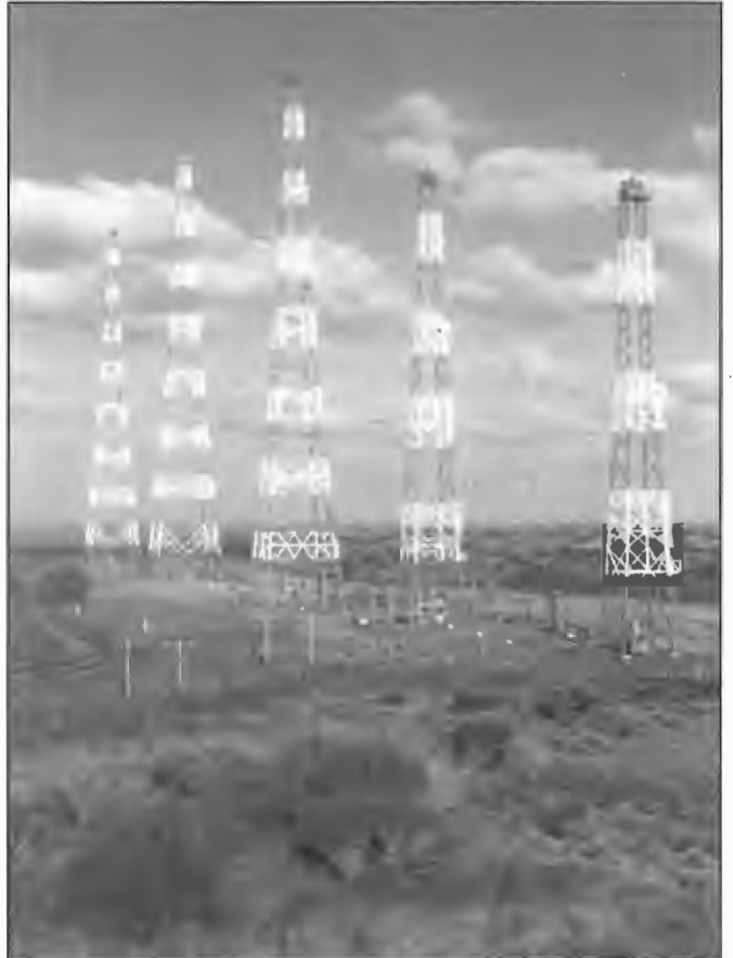
Aerial support towers Radio Australia, Carnarvon erected 1975. The structures designed by Brown Boveri Co., supported four aerial systems each of HR4/4/0.5 configuration. The tallest towers were 100 m high and supported the 6,7,9 MHz band aerial system.
