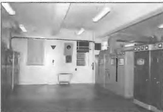
NBS transmitting centre, Canberra. (Left) 2CN 2 kW transmitter. (Far right) 2CY STC 10 kW main transmitter. (Near right) 2CY AWA 2 kW standby transmitter. Station 2CY began operation on 23 December 1938 followed by 2CN in 1953. The 10 kW STC transmitter was installed in 1964. As at 1992, the 2 kW AWA transmitter was being used for Radio for Print Handicapped Service.
