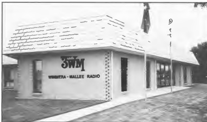
Administration and studio building 3WM Horsham, erected 1982. Senior Technician Bruce Lees.
