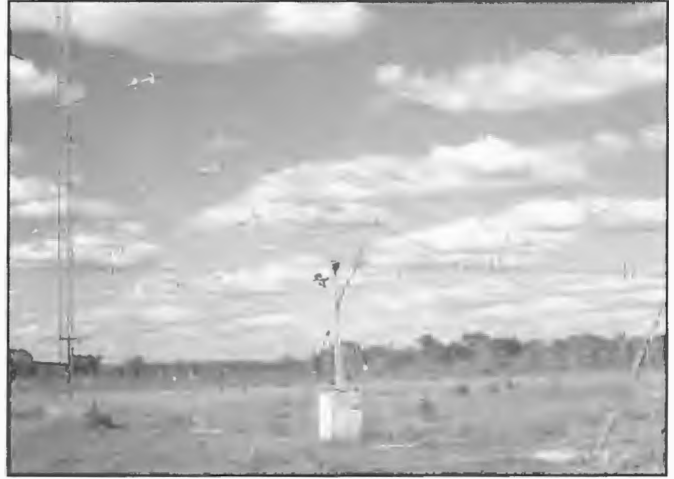
Vertical incidence log periodic aerial provided at High Frequency Inland Service stations located at Katherine, Tennant Creek and Alice Springs in Northern Territory during 1986. Dipole elements were so positioned from a support catenary that the active elements were always a quarter wavelength above ground. Senior Lines Officer, Jim Finch.
