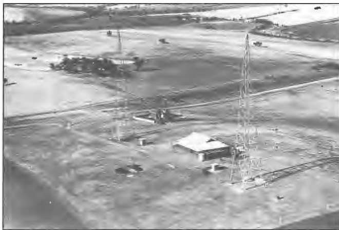
Station 5CK Crystal Brook began operation on 15 March 1932 with a 7 kW water cooled transmitter feeding a multiple tuned flat top Alexanderson type aerial supported by two 56 m towers. A house was erected on the site for the first Officer-in-Charge Bill Whisson.
