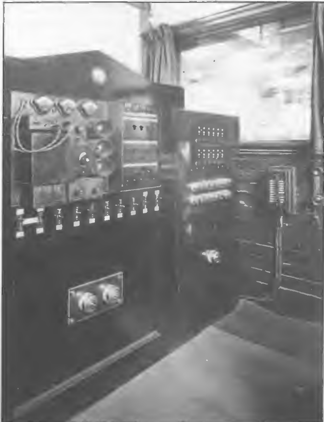
Original equipment and power control racks 3LO control room 1924. The Western Electric line amplifier was a three stage amplifier employing WE type valves. Meters and patch cords enabled anode and filament currents to be measured. Rheostats enabled each filament current to be adjusted to correct value. A and B batteries for filaments and anodes respectively, were located in the battery room but C batteries were located in a grid battery box alongside the amplifier on the rack. A 22 step potentiometer controlled the output level of the amplifier.
