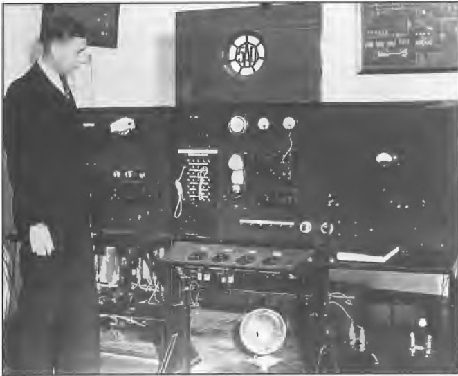
Program input equipment and control centre 5AD Adelaide 1936. Chief Engineer Don Gooding making adjustment. He was Chief Engineer from 1931 to 1961. The station began operation on 2 August 1930 and the control room equipment included a four channel input audio mixer together with turntables for playing discs from the control room.
