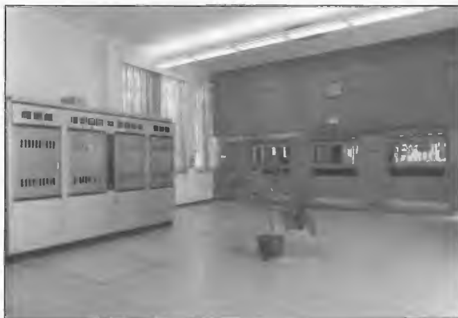
AWA BTM10 standby 10 kW transmitter (left) and STC 55 kW transmitter 3WV Dooen. The 10 kW unit was originally installed as the main unit in 1959 and the 55 kW model began operation on 31 August 1960. Over the years, the building had suffered a number of structural problems due to soil movement and in 1988 a new building was erected and a 55 kW solid state transmitter installed.
