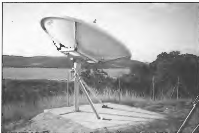
Acesat Satellite Corporation Pty Ltd receiving dish beamed on Ominicast satellite for programs for Totalisator Administration Board of Queensland, Thursday Island FM transmitter. The station was one of sixteen Queensland country stations commissioned during 1993 for the TAB. Dishes for the network were supplied as 3 or 3.7 metre diameter.
