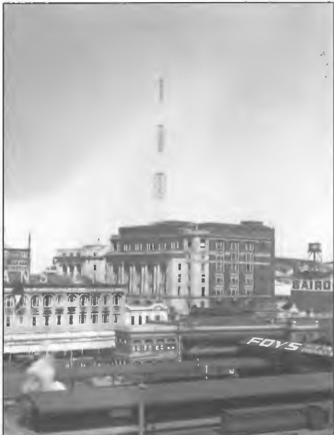
Self-supporting 60 m tower on roof top of Perth GPO employed as the radiator for 6WN which went to air on 12 October 1938. The feeder linking the 500 watt transmitter to the aerial was an 80 ohm concentric type. During the War years, the tower was dismantled and the transmitter shifted to another site.
