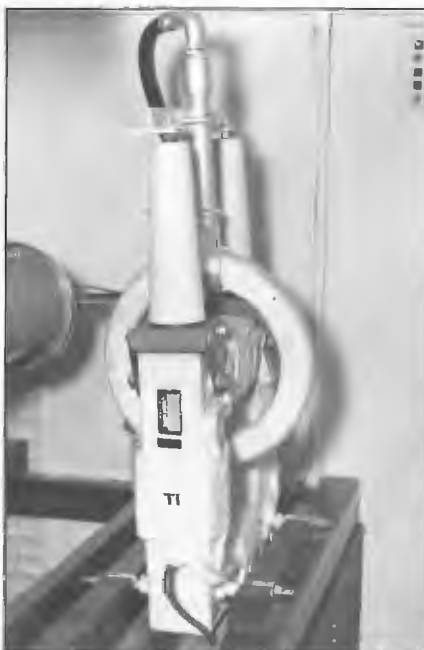
Mast lighting transformer designed for use at base and sectionalising point for 5CL/5AN Pimpala 172 m radiator 1961. It was designed and developed by Bland Radio Ltd, Adelaide to specifications prepared by Bill Gold. It was an alternative arrangement for feeding AC power wiring through the tubing of an inductor or via RF chokes. The company subsequently supplied units for use at other NBS stations and also Commercial stations in other states.
