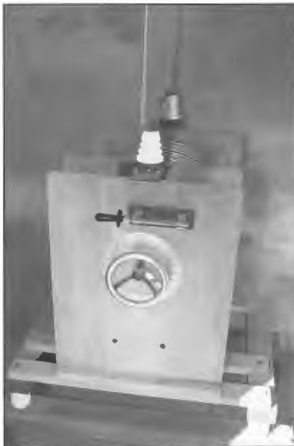
multiple wire aerial. Feeders were cage types and terminated in variable inductors located in tuning huts near the support towers.
