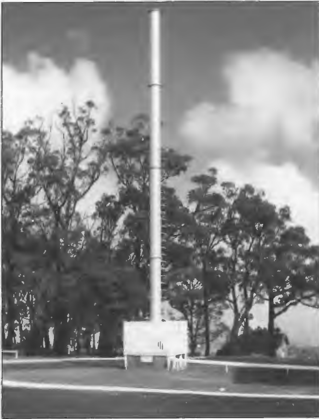
A 17 m pylon type radiator comprising slotted line sections provided for the ABC FM service Adelaide in 1951. It was originally installed at Mt Bonython but later transferred to Mt Lofty, the site of the present National TV and FM services. It ceased to be operational when the FM mono service was closed down in 1961 but in later years served as a standby when the FM Stereo service commenced. Engineers associated with the design and commissioning were Frank Norman and Frank Brownless.
