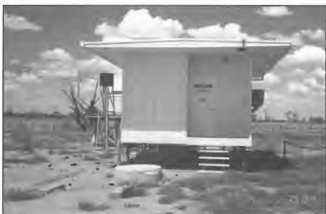
Typical prefabricated Logan type building provided at National Broadcasting Service stations from the late 1980s to house 10 kW Nautel Amphet solid state transmitters. This building housed the 4QL Longreach facilities.
