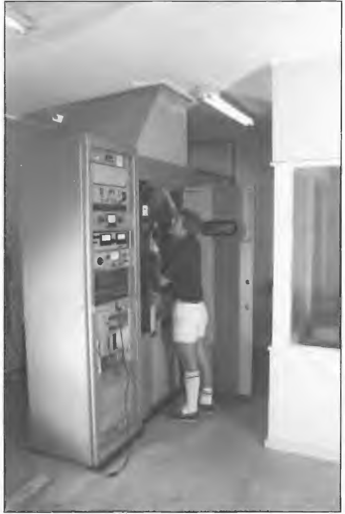
Alan Hubbard making adjustment to AWA BTM2 emergency transmitter, Berry Springs. The transmitter provided 2.5 kW into a top loaded radiator and was set up on the same frequency as NBS station 8DR. David Young was installation Engineer.
