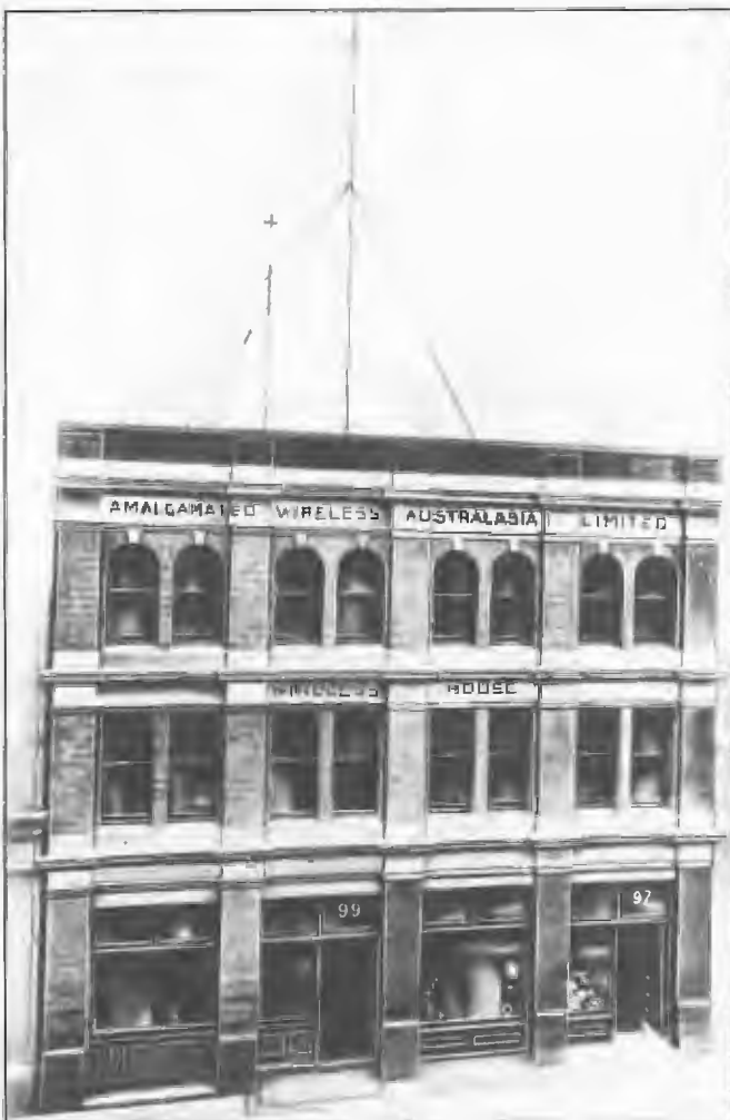
Wireless House, 97-99 Clarence Street, Sydney, the first headquarters and factory of Amalgamated Wireless (A/Asia) Ltd following formation of the company in 1913. In 1922, production activities were transferred to new premises at Knox Street, Sydney. The multiwire roof-top aerial was employed with the first public demonstration of broadcasting to members of the Royal Society in 1919. Technical Director and General Manager, Ernest Fisk.
