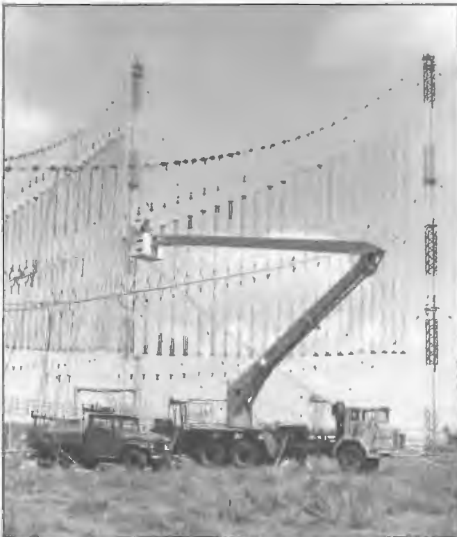
Method of gaining access to the dual plane log periodic aerial system installed in 1969 at Radio Australia, Cox Peninsula. The aerials were designed and manufactured by Complementi Elettronici S.p.a., Italy and installed by RCA (Australia) Pty Ltd. It was the first time the design had been employed to handle 250 kW input for International broadcasting purposes. RCA Engineer, Ross Burbidge.
