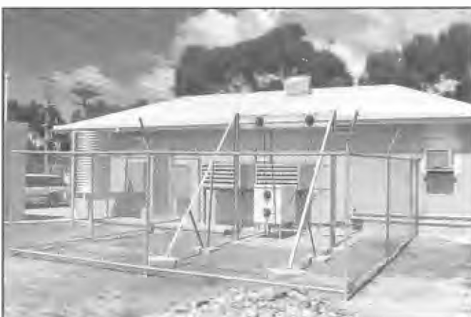
Transmitting station building 3WV Dooen, erected 1988 to replace original 1936 building.
