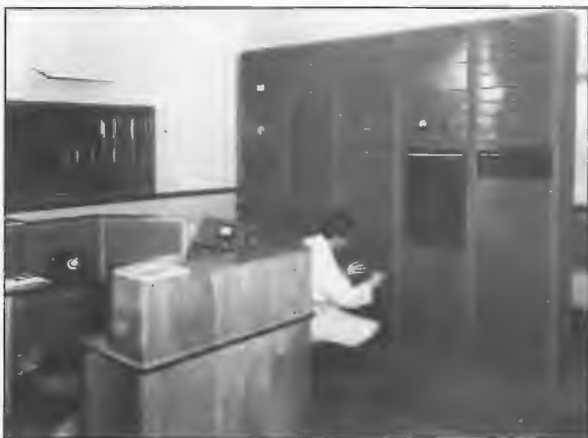
Control room Adelaide Street studios 4BC Brisbane circa 1937 showing AWA control panel, rack equipment and patch panels typical of the period, Station 4BC was the first Commercial station to go to air in Brisbane when it employed a temporary transmitter on the roof of a building at 43 Adelaide Street where the studios were also located. On air date 16 August 1930.
