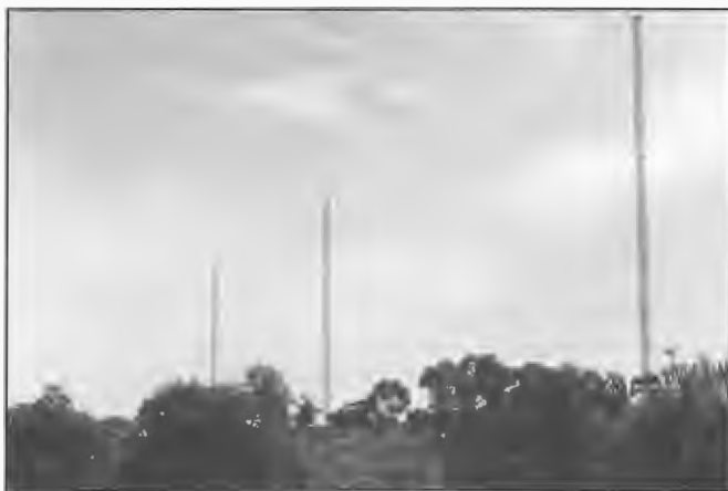
Main 6 and 9 MHz aerials employed at National station VLW Hamersley for ABC HF Inland service. Each aerial comprised dipoles and reflector curtain suspended by 40 m guyed lattice steel masts. The service was closed down during 1994. Station Officer-in-Charge, Murray Little.
