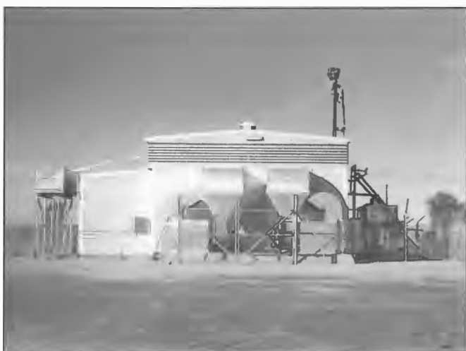
Transmitting station building for HF Broadcasting Service Northern Territory. Identical buildings were erected at Alice Springs, Tennant Creek and Katherine, 1986.
