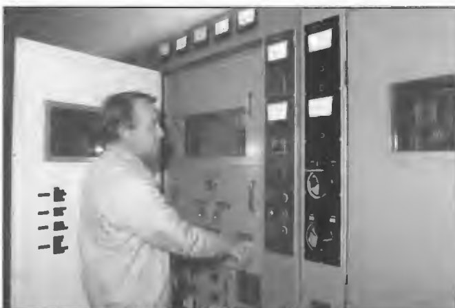
Murray Little, Officer-in-Charge adjusting one of the three VLW transmitters associated with the HF Inland service based at Hamersley near Perth. The service operated with two 10 kW and one 50 kW transmitters, broadcasting on three frequencies. The service was closed down during January 1994.
