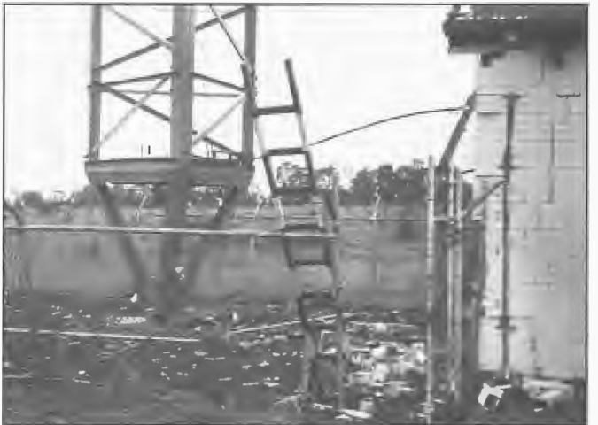
Damage to base of 2BL/2FC 230 m high dual frequency radiator Sydney as a result of vandalism in 1969. A charge of high explosive was fired at the base and destroyed the base insulator causing the 50 tonne mast to drop 60 cm. The aerial coupling equipment building was extensively damaged and 17 guy insulators were damaged by shock impulses transmitted to the structure.
