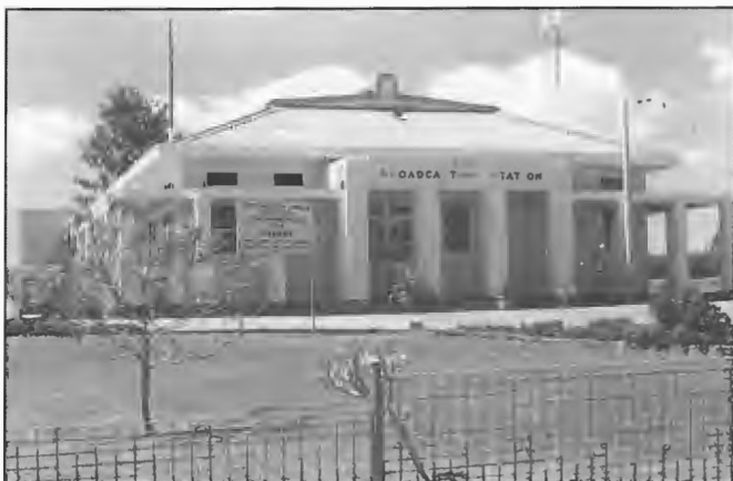
Transmitting station building 2NR Lawrence, erected 1936. First Officer-in-Charge E.J. Halcrow.
