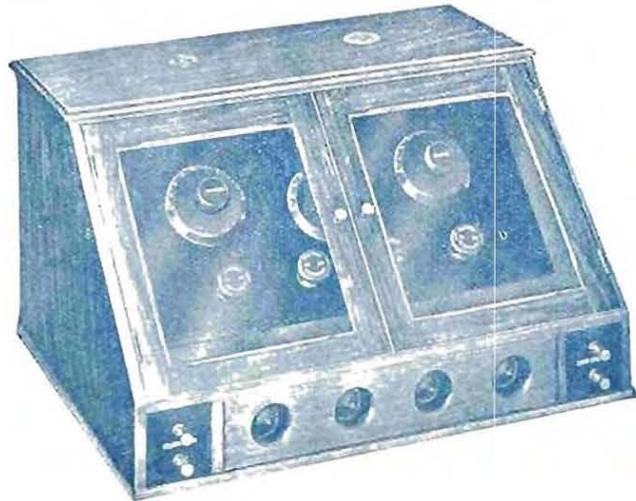
The two illustrations on this page depict the New System T.M.C. Four Valve Set. It consists of one high frequency, one rectifying and two note magnifying valves. Has a separate filament control for each valve. Gives excellent reception from Broadcasting Stations, and may be used in conjunction with a TrueMusic Loud Speaker with splendid effect.
