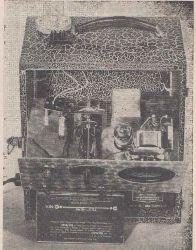
These close-up views provide all the detail necessary for the layout and assembly of the transceiver. Note the method of mounting the 76 horizontally to ensure short leads, and the tuning condenser extension shaft employed for the same purpose.
