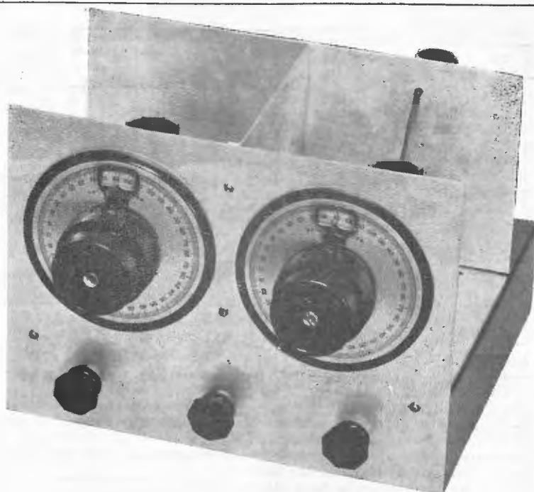
**T**HIS three-valve battery shortwaver was designed primarily for simplicity of construction and operation, but also for high efficiency and low cost. The parts used are all standard; in fact, many set-builders will have quite a few of them on hand already.
