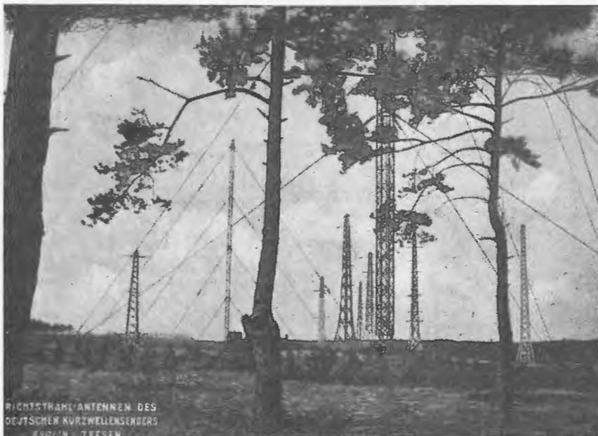
A view of the directional aerial arrays used for the German world shortwave service. The interval signal used by all stations consists of eight notes of an old German folk song.
