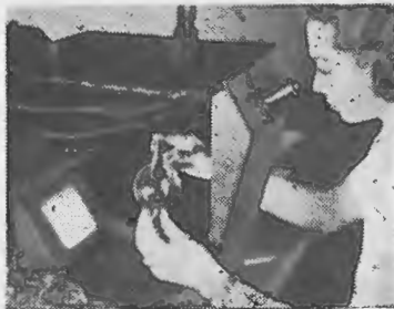
Polariscope is here used to inspect glass bulbs for flaws or strain which may occur during the shaping operations
