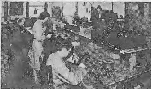
At left: Portion of one of the assembly lines at the Magrath factory. Aegis coils and I.F.'s being made.
