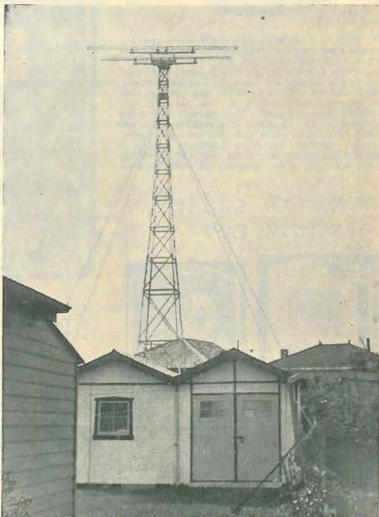
28 M/cs. Beam Array of VK2AKR, Lidcombe, N.S.W.
