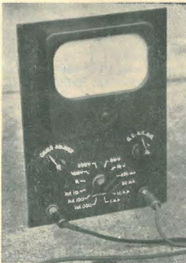
The multi-meter which is assembled from the kit.
