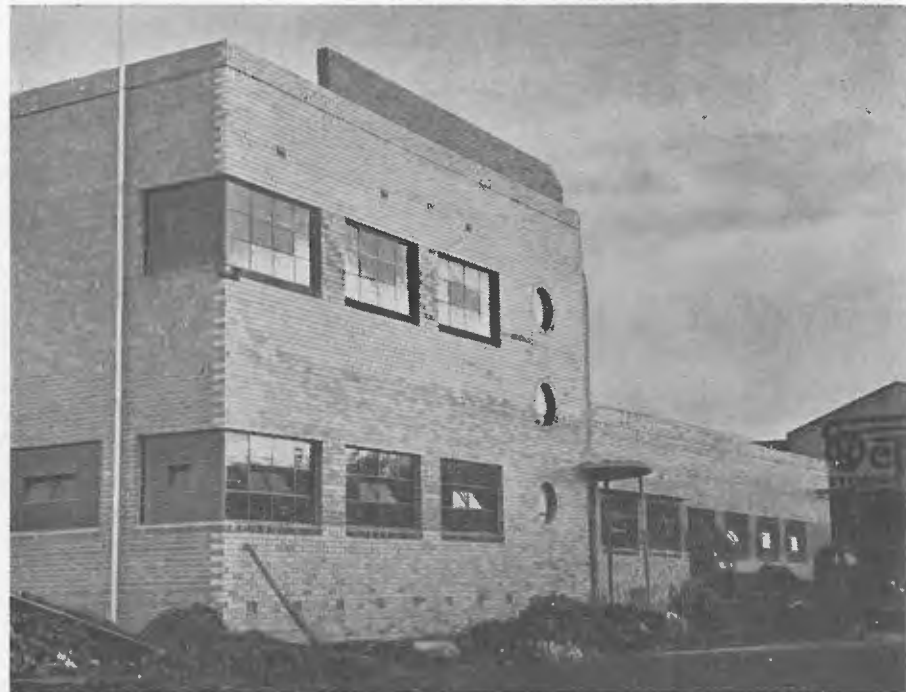
Rapidly nearing completion is the new T.E.P.L. factory, Doonside Street, Richmond, Victoria. Illustration shows the modern and distinctive lines of this up-to-date factory for the manufacture of broadcasting equipment and associate products.
