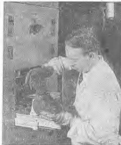
A bakelite preform after it has been heated for approx. 40 seconds. Note the plasticity of the preform and the uniformity of the heating right to the centre of the powder.
