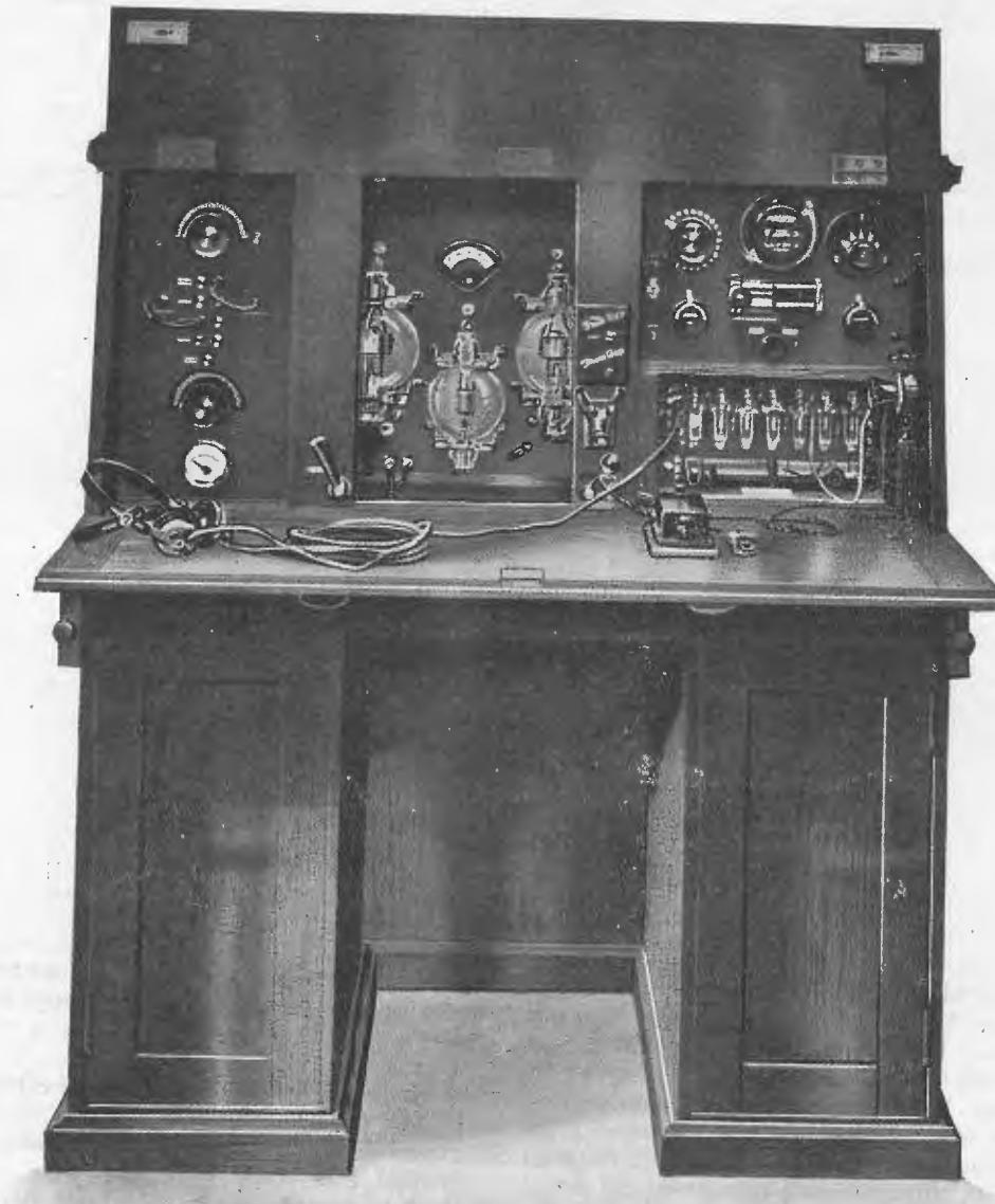
Half-K.W. Wireless Telephone Telegraph Transmitter and Receiver, Manufactured by Marconi's Wireless Telegraph Co., Ltd., London, and Amalgamated Wireless (Australasia) Ltd., Sydney.
