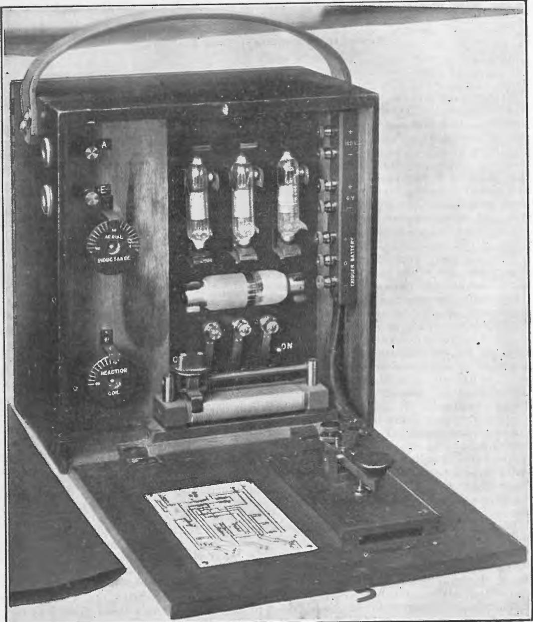
Two Watt Valve Transmitter, Manufactured by Amalgamated Wireless (Australasia) Ltd.
