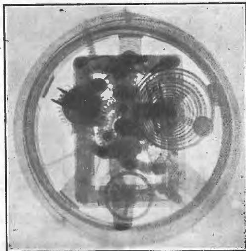
Fig. 3.—Radiograph of an alarm clock.
