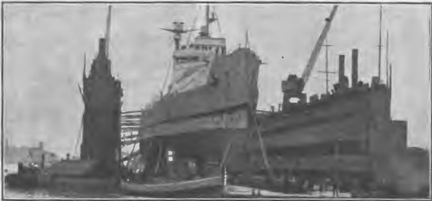
WARSHIP UNDER REPAIRS AT A FLOATING DOCK.
