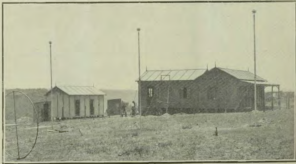
The main operating room and store at 2FC. One of the hoops used in the large aerial is in the foreground to the left.
