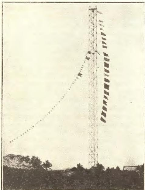
The 280 ft. mast at Townsville Radio. It is a portion of one of the masts captured from the Germans at Bitu Paka, in 1914. Townsville handles the bulk of the traffic to the Mandated Territory, and to the Islands. The station is fitted with a
