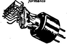
2. The control grid is next added being wound at right angles to the filament
