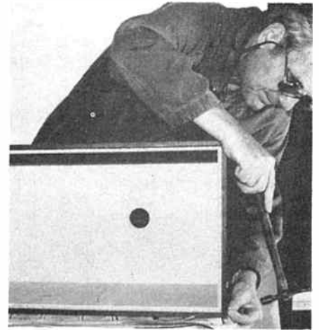
Hammer panel pins in the last corner to hold the cabinet together until dry.
