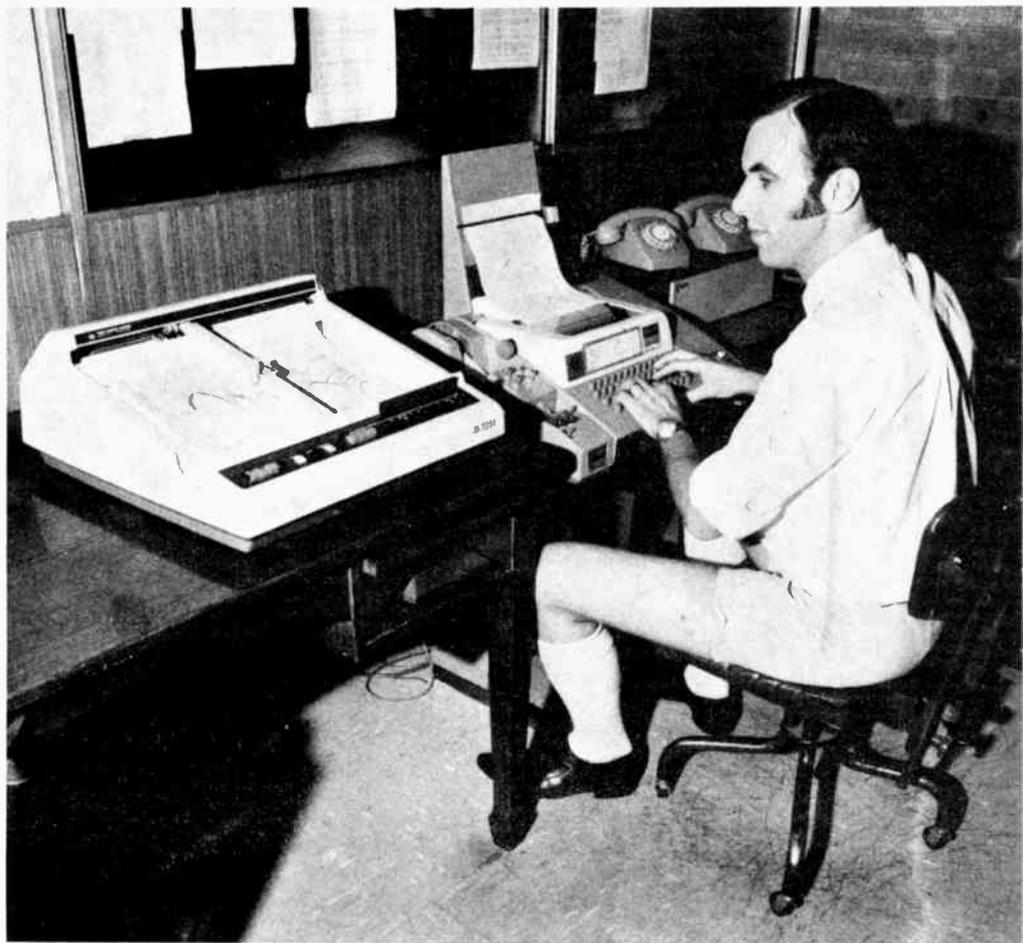
*Don Craig of AWA's Engineering Products Division uses computer terminal and HP 7200A Graphic Plotter to determine polar response of loudspeaker columns.*
