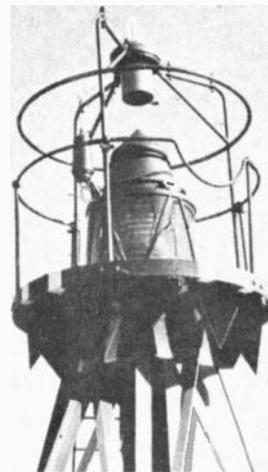
The distinctive racon signal clearly shows the position of a seamark or landmark on a ship's radar screen by providing its range and bearing. This is useful when the landmark or seamark is not visible, is indistinct, or cannot be discriminated from other echoes.
