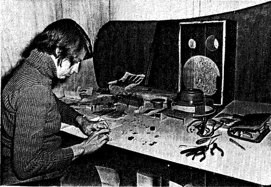
Jan commences assembly of the first of the two loudspeakers — note the massive 14" diameter JBL woofer.
