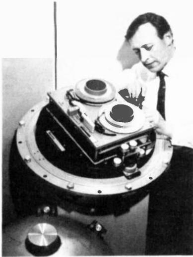
This underwater data centre — produced by GEC-Marconi — accepts inputs from almost any oceanographic instruments and records time-correlated data in computer retrieval form on magnetic tape.
