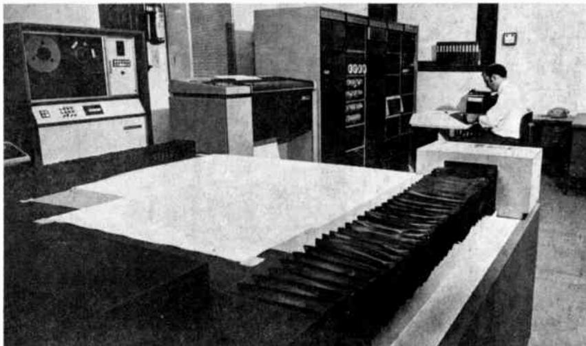
The modern minicomputer has dispelled many of the traditional notions about its limitations, and this is well illustrated by the new PDP-11/45 machine being used by the N.S.W. Lands Department for surveying and cartographic work.
