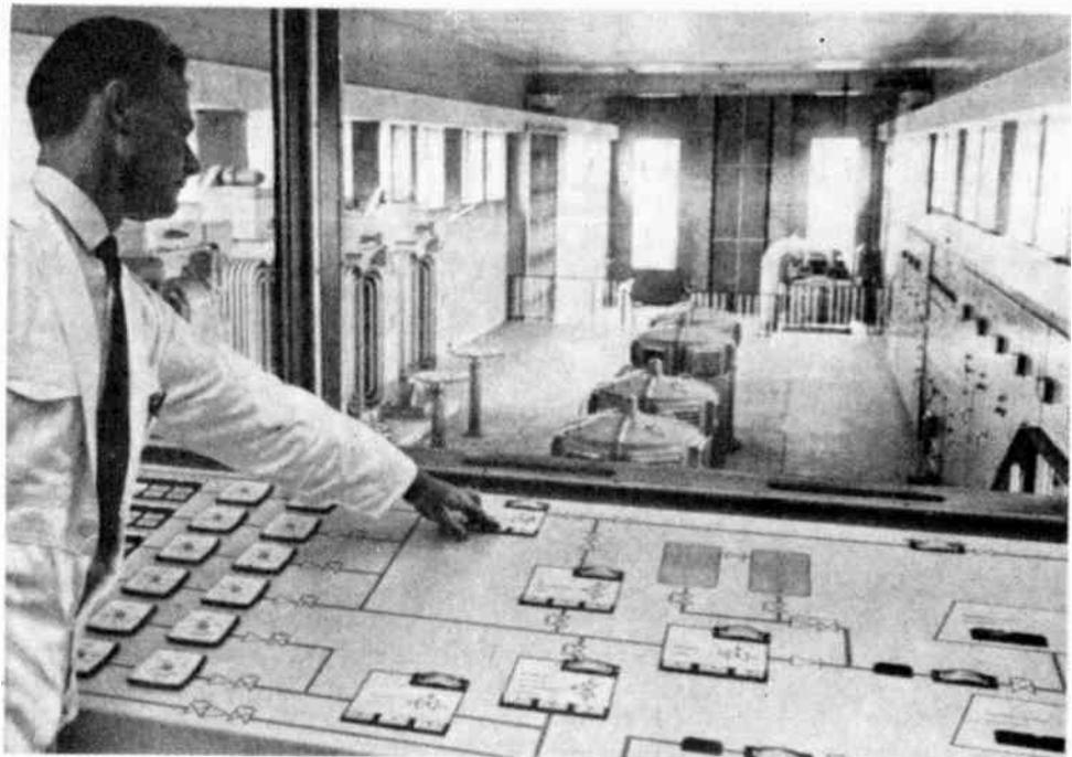
Fig. 10. Human engineered control panel of computer-controlled water distribution station — controls are laid out in the mimic diagram.
