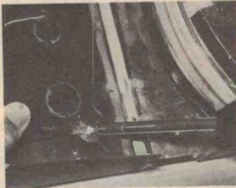
**1.30pm** "Resolder a 7/036 earth to sheet metal — LP gas flame would work, but too much risk of heat damage to PVC cable. The Superspeed iron produced its full 150 watts and did the job".
