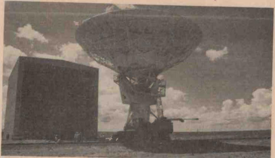
A special transporter vehicle was constructed to carry the huge antenna assemblies to their sites once their construction was completed. Above is antenna No.1 on the transporter, July '75.
