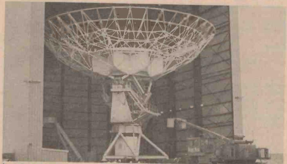
An unfinished antenna in the antenna assembly building — also specially built for the construction of the antenna assemblies. Some idea of the size can be gauged from the small figures visible at the base of the antenna, adjacent to the transporter (right).
