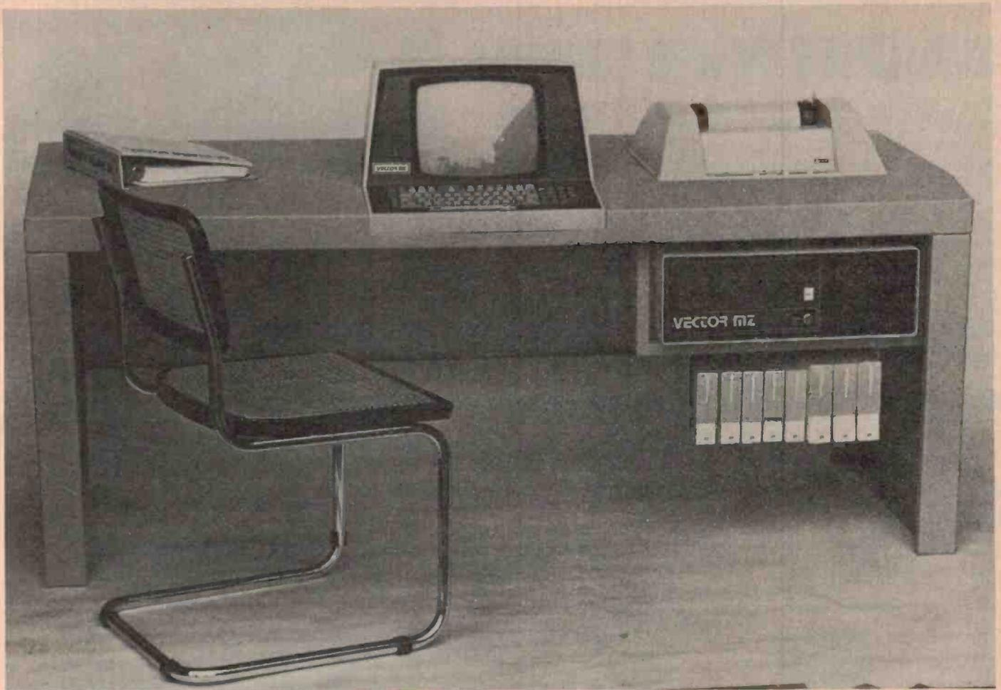
The 'Memorite' word processing system has the same basic hardware as the System B but can be used with a Diablo or Qume printer to provide good quality copy suitable for photocopying or instant printing. Software for the system is contained in ROMs and the dual mini-
