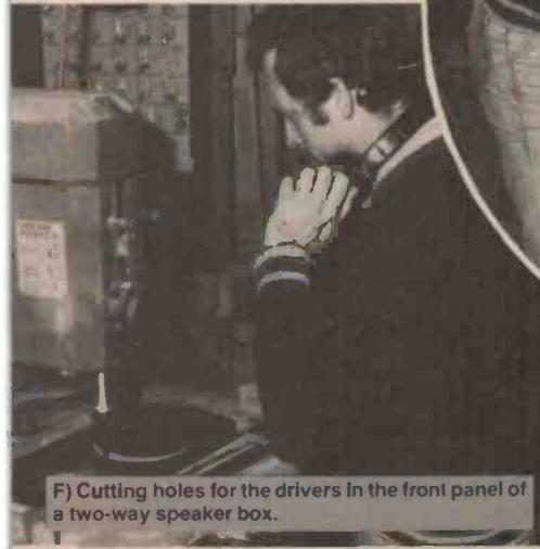
F) Cutting holes for the drivers in the front panel of a two-way speaker box.
