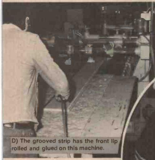
D) The grooved strip has the front lip rolled and glued on this machine.
