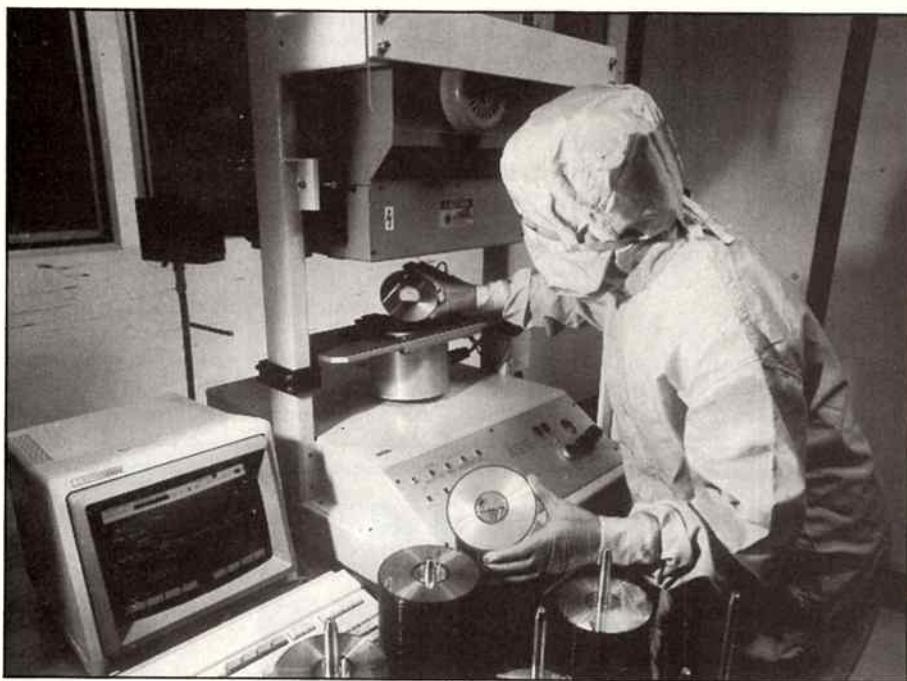
*Using the laser scanner to check for quality.*
