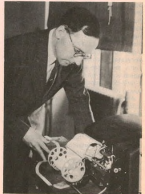
EDSAC, one of the first electronic digital computers, built at Cambridge University in 1949. The shot at right shows Dr. M. V. Wilkes, leader of the team which produced the machine. It used more than 3000 thermionic valves. The name "EDSAC" stood for electronic delay storage automatic calculator.
