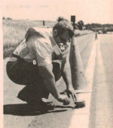
View at left shows Kenney using an oscilloscope to analyse field data in the laboratory. Above, Kenney setting up a transducer at the edge of a heavily travelled highway.
