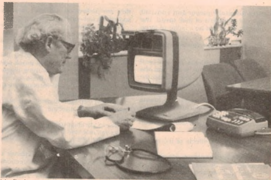
Medical consultation is an obvious use for the TV telephone. Here a doctor uses the experimental Dutch network to discuss a chart with a colleague. The chart, on the desk, is reproduced on the screen. Note the angled mirror in front of the camera.
